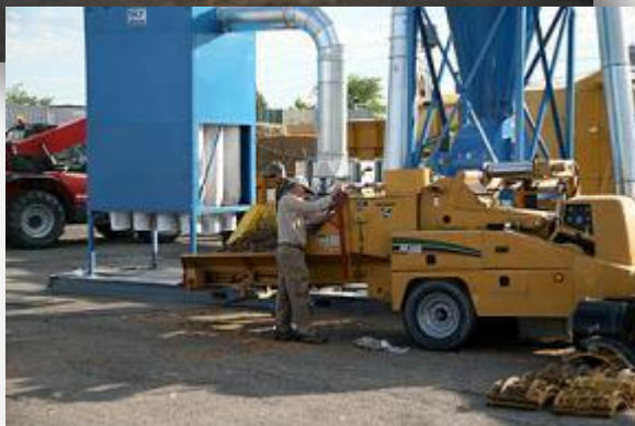
Pneumatic transfer system (blue, left) supplied air flow through the grinder, increasing capacity by a factor of two.
