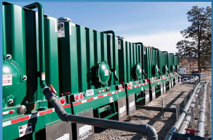
Chromium-contaminated groundwater was stored in tanks prior to treatment.
