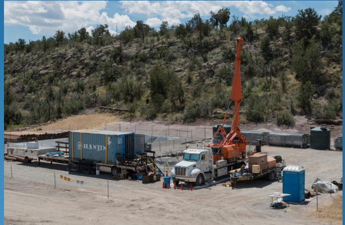
A crew drilled CrEx-1, the project's first extraction well for hydraulic control.
