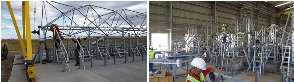
Figure 16: Installation of OP20 fixture station over existing trench in the foundation (left) vs. elevation of the fixture assemblies to avoid installation of trench in the foundation – Xina (right)
