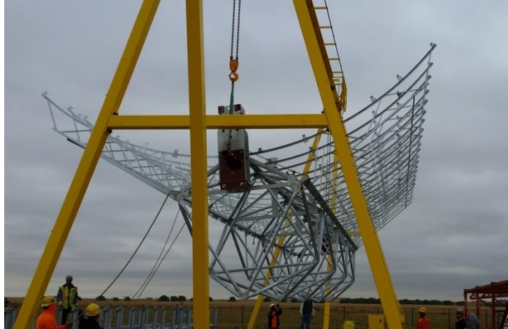
Figure 22: Module suspended from crane with flipper at each end
