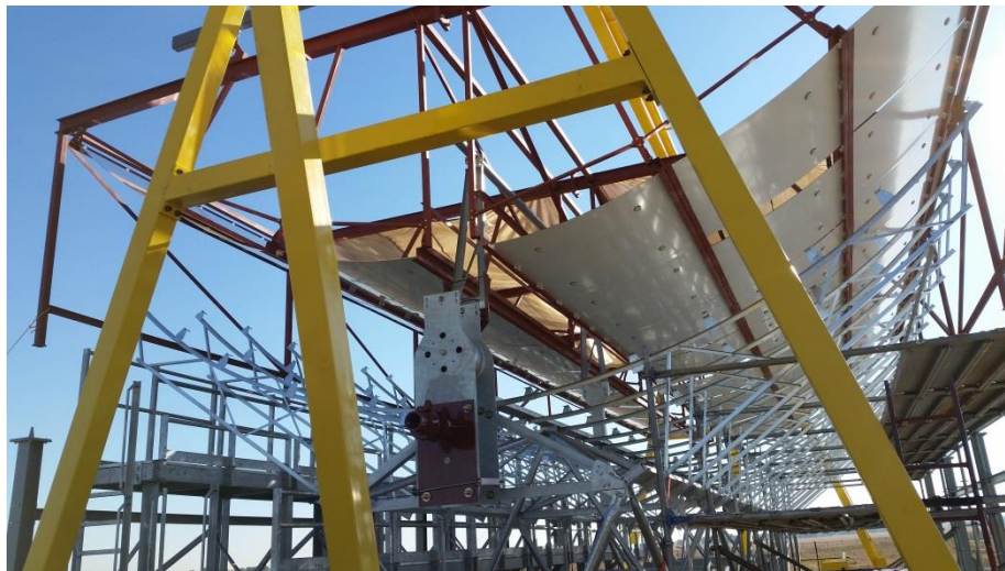
Figure 23: Mirror rack being lowered over SpaceTube module in OP30 station
