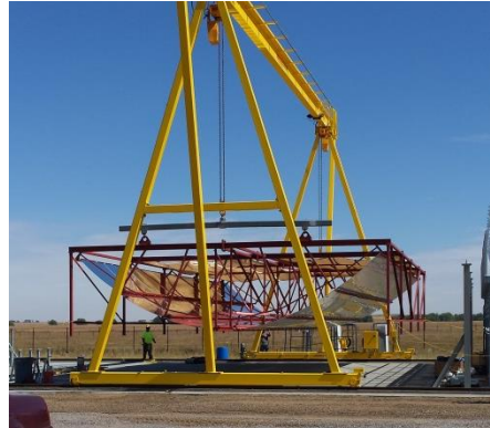
Figure 17: Gantry crane used for the SolarMat demonstration Prototype
