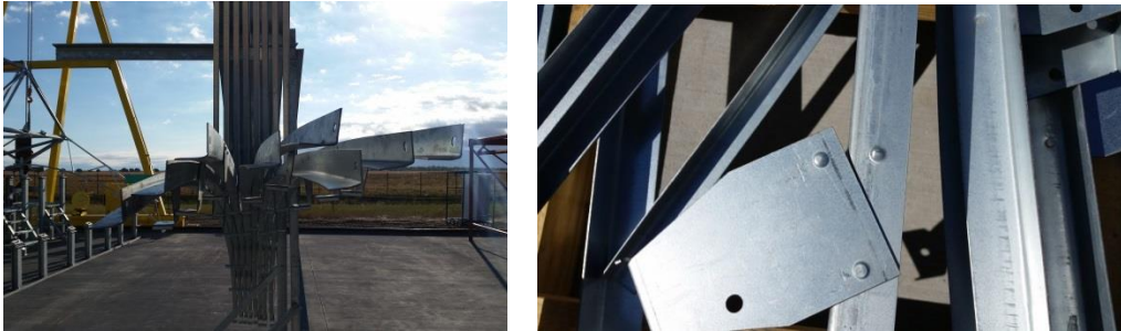
Figure 26: (left) View of arms on the transportation cart (note: the top chord should align on all arms. (right) Non Typical self-piercing rivet joint at the mirror support bracket (note; the SPR did not penetrate the top layer - indicating incorrect joint design or implementation I.e. setting pressure, speed, etc.)
