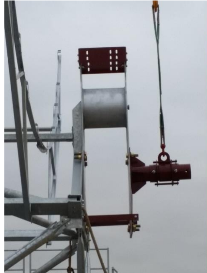
Figure 9: Flipper attached to the TTA/ETW assembly. Shown while module is supported by crane (typical OP20-OP30 transition (note: excessive deflection in the TTA plates))
