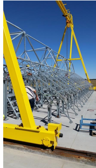
Figure 27: Module nearing completion on OP20 station
