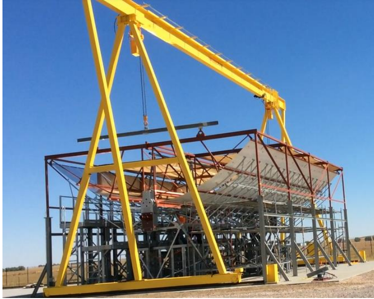
Figure 31: Mirror rack resting in mirror installation position
