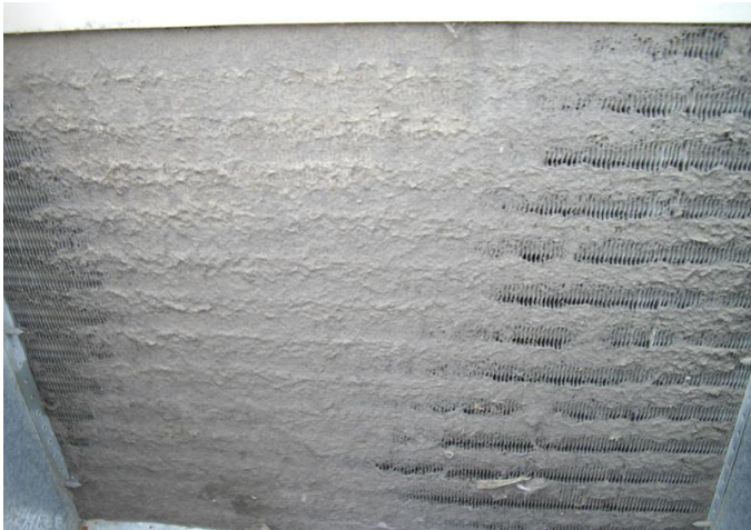
Fouling of evaporator coil 3
