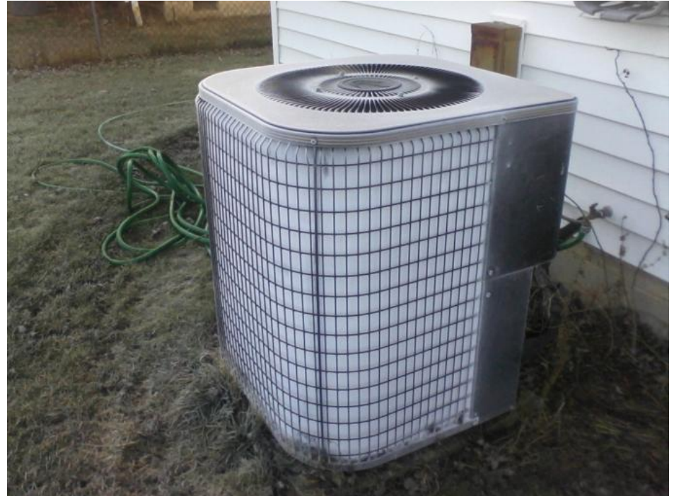
Frosted evaporator in cold climates 5
