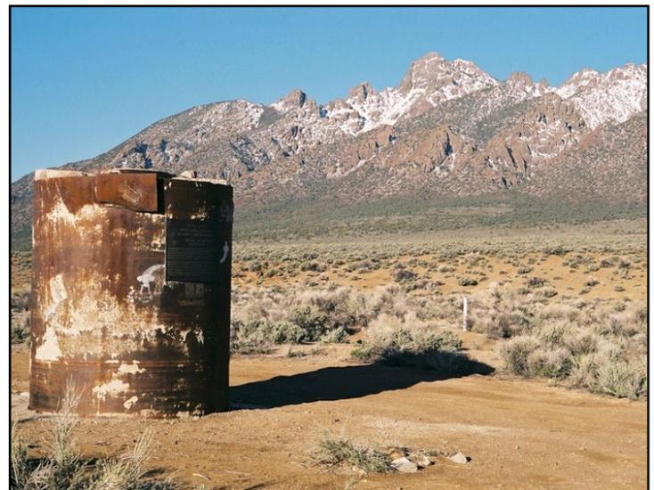
Surface casing for UC-1 (emplacement borehole).
