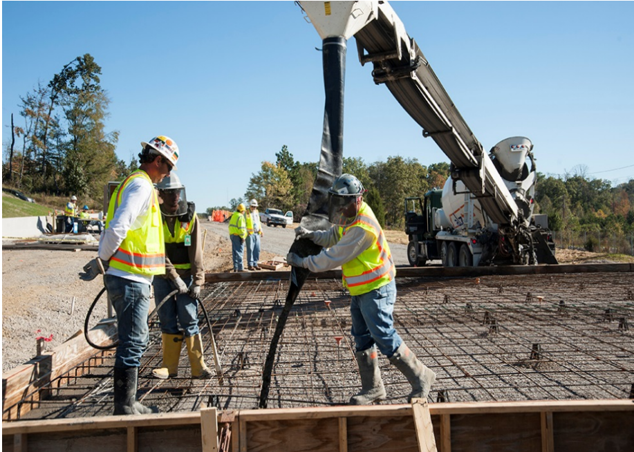
CNS/Northwind Portal 19 Concrete Pad Placement
