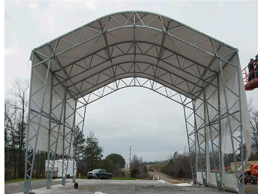
CNS/Northwind Erecting Portal 19 Canopy Structure
