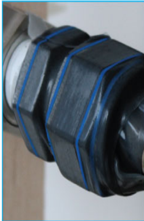
Hydrogen Leak Detected
