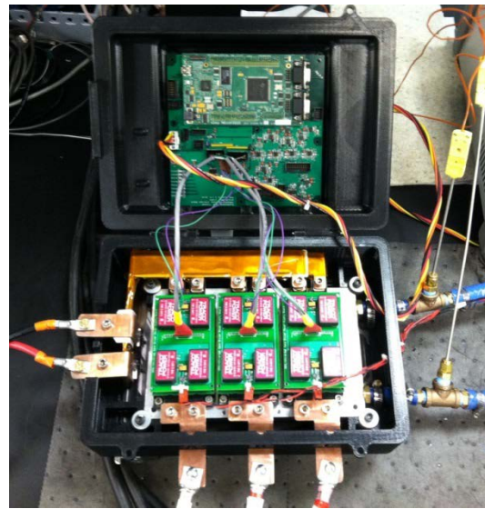
(b) Assembled inverter
