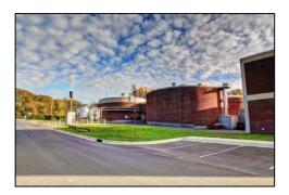
The City partnered with Unison Solutions, a Dubuque-based biogas conditioning manufacture, to design a system that would shift from previously-utilized incineration technology to innovative anaerobic digestion. The plant, completed in 2013, is the first in Iowa designed to meet EnergyStar requirements. The switch enabled the facility to harness biogas for digester heating and electricity generation.
