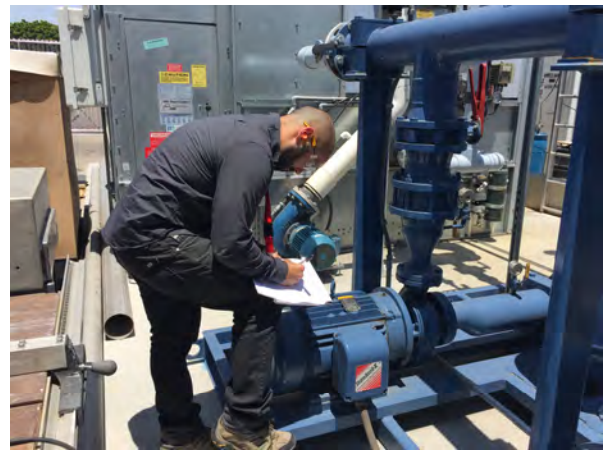
An Industrial Assessment Center (IAC) student examines pumps at an industrial facility. Photo courtesy of the San Francisco State University IAC.
