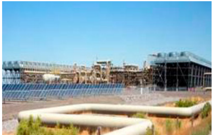
Enel Stillwater hybrid geothermal-solar facility in Fallon, Nevada. Source: Enel Green Power North America
