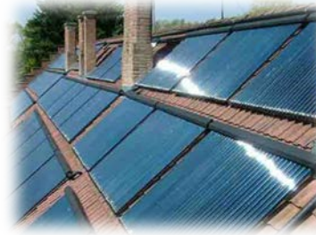
Solar Water Heating
