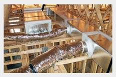
The insulated ducts were installed close to the ceiling and were well sealed.
