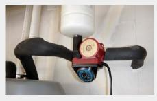
A simple approach is to add a circulation pump that senses a request for hot water. The main hot water must form a loop.
