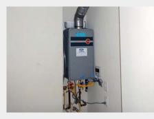
Instantaneous water heaters, even tanktype heaters, can be distributed among water-use zones to minimize water and energy waste.
