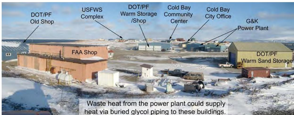
The buildings in each scenario will receive heat from an insulated, buried district heating loop that delivers waste heat from G&K's diesel generators. Piping lengths vary depending on the scenario. Please refer to the Moolin report for piping lengths, building heating loads, waste heat production and system layout.
