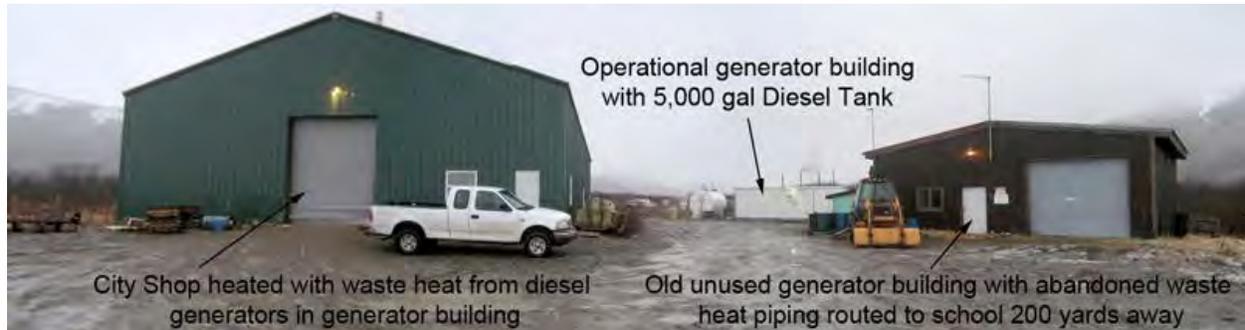
During the site visit an old waste heat recovery system was found at the Old Generator Building that includes a 3" HPDE piping loop to the school approximately 200 yards away. The pipe was insulated with spray foam only on the top side of the piping, with no other protection from the environment.
