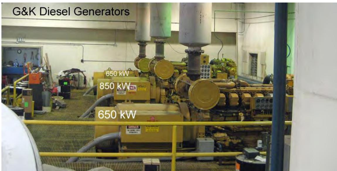
The generators were installed in 1987 and now have between 67,000 and 79,000 hours of operation on them. The generators are well maintained and each one has been rebuilt at least twice. G&K expects them to have a usable life of 150,000 hours. Replacement cost for a single generator is over \$300,000. Below is a summary of the generators and their status.
