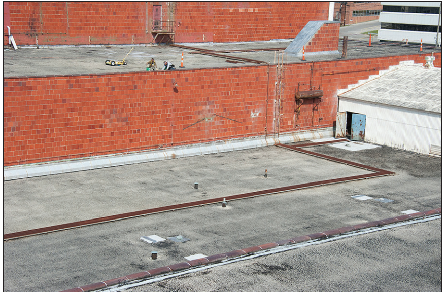
Alpha 4 roof repairs
