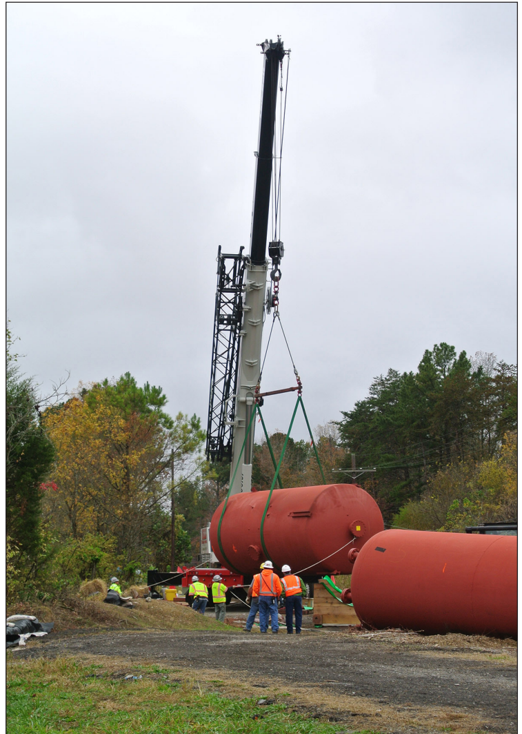
Abandoned tanks at the Y-12 Complex
