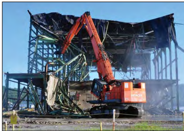
Demolition of the K-31 Building at ETPP was completed in June. K-31 was the fourth of five gaseous diffusion buildings to be demolished in Oak Ridge.
