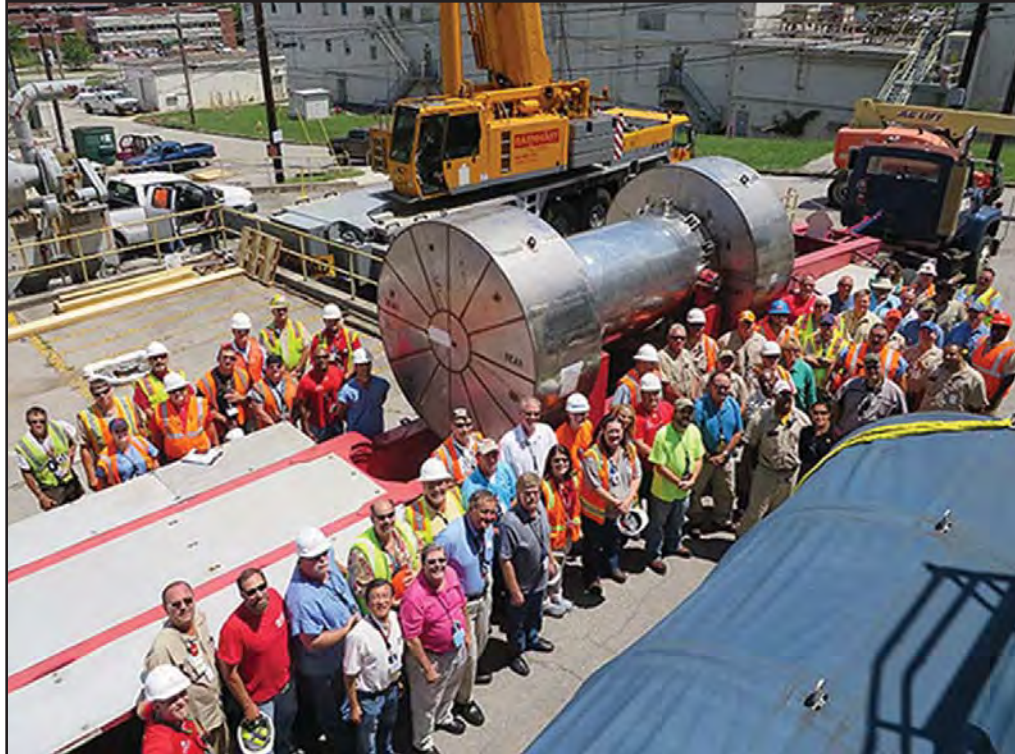
Workers celebrate the successful removal and packaging of radioactive components from the Oak Ridge Research Reactor pool. The components were shipped to Texas for disposal.
