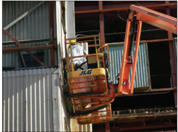
Transite paneling removal.
