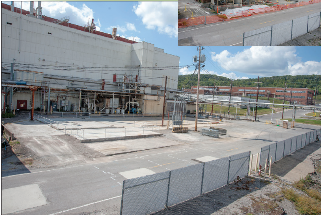
Building 9808 before demolition (right) and after (below).
