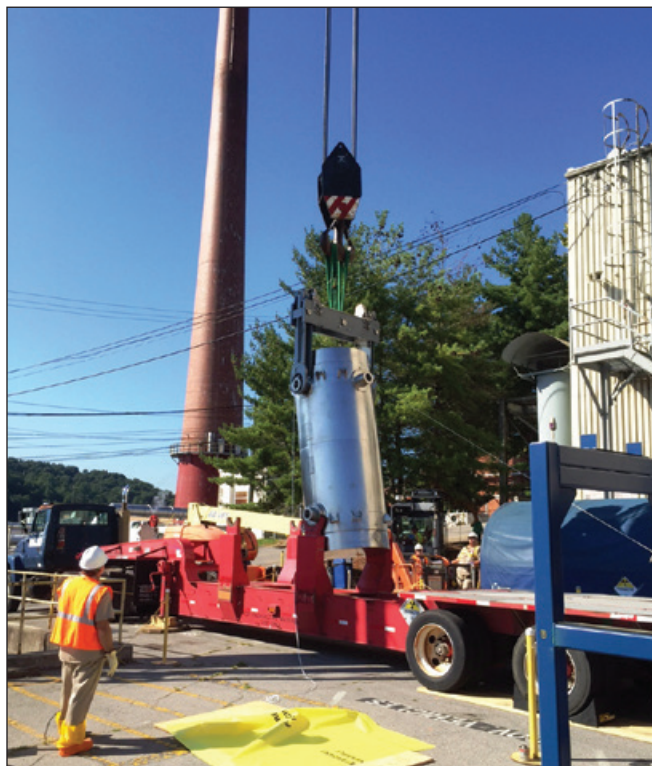
Workers load cask onto transport truck.
