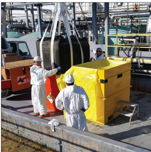
The dewatering bag is being moved from its yellow frame into a shipping container.
