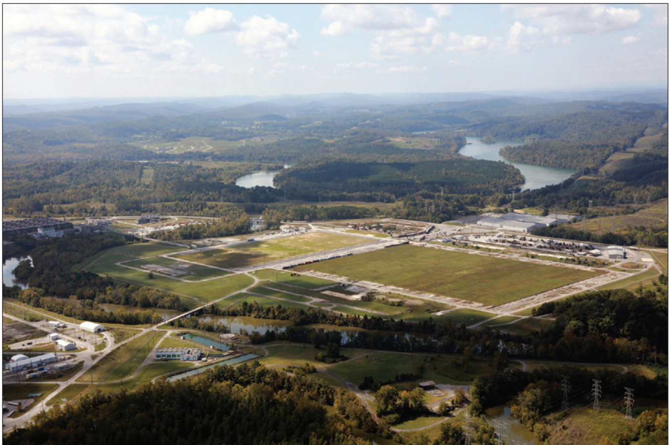
Demolition of K-31, which was preceded by demolition of K-33, has created a large land parcel available for private use.
