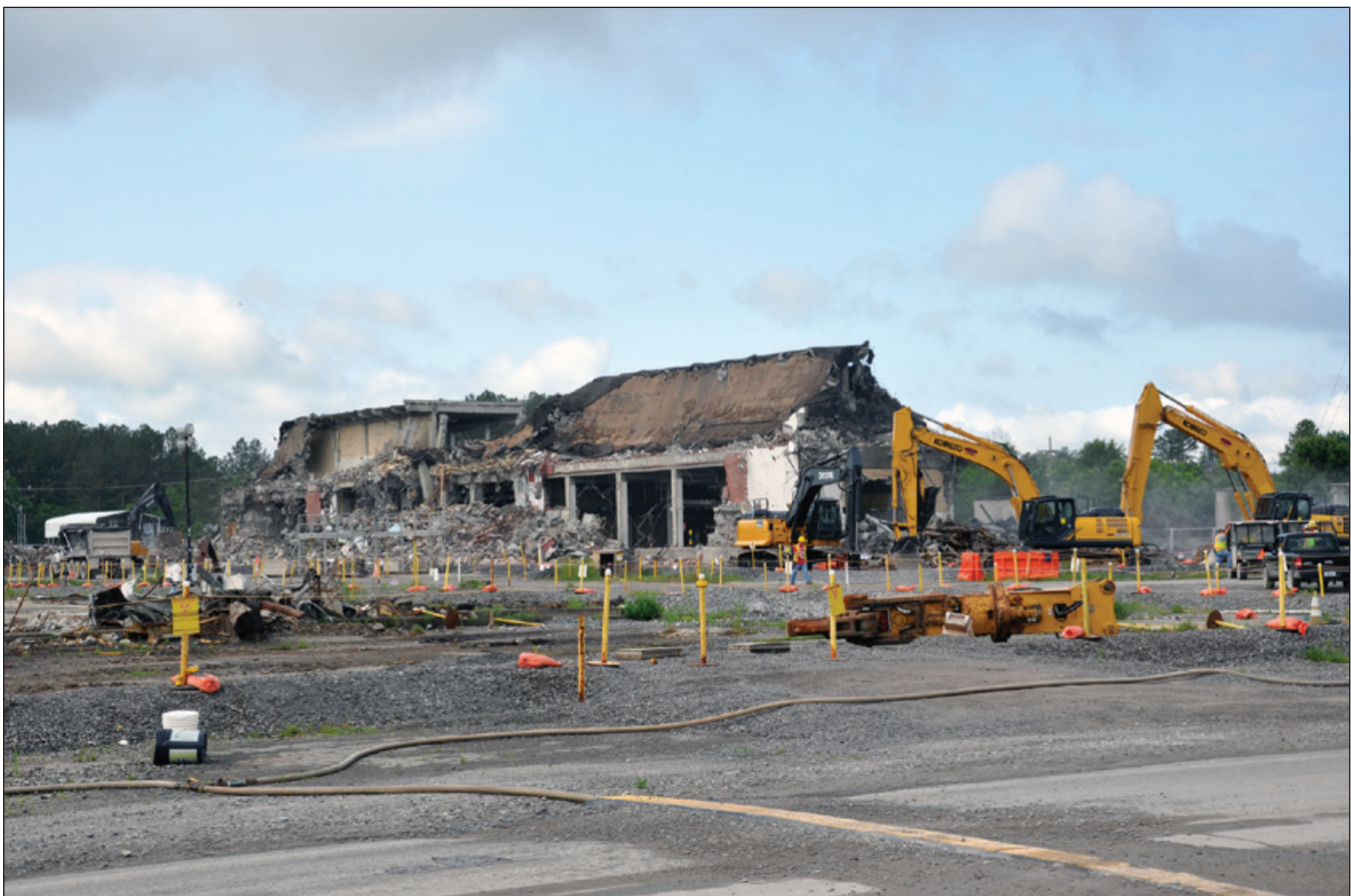
Demolition of Building K-761 Switch House.
