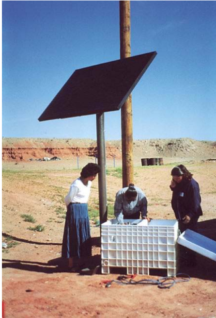
Sandra Begay-Campbell with two Navajo electrical technicians checking an NTUA PV system in the Kayenta District, Arizona.
