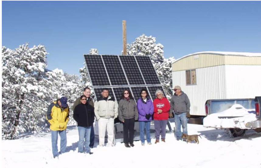
New NTUA Off-Grid Photovoltaic (PV) Hybrid Unit
