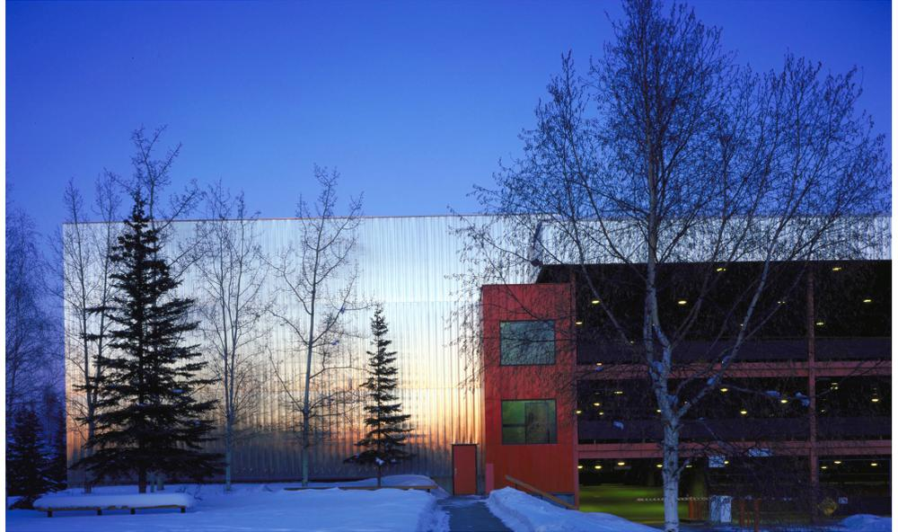
The Northwest/Arctic Region branch of the GSA improved safety and energy efficiency in their Fairbanks Federal Building parking garage used by federal employees and a lower level used by the U.S. Marshals and the District Court. A 74% savings was realized by replacing 220 HPS fixtures with 220 LED fixtures.
