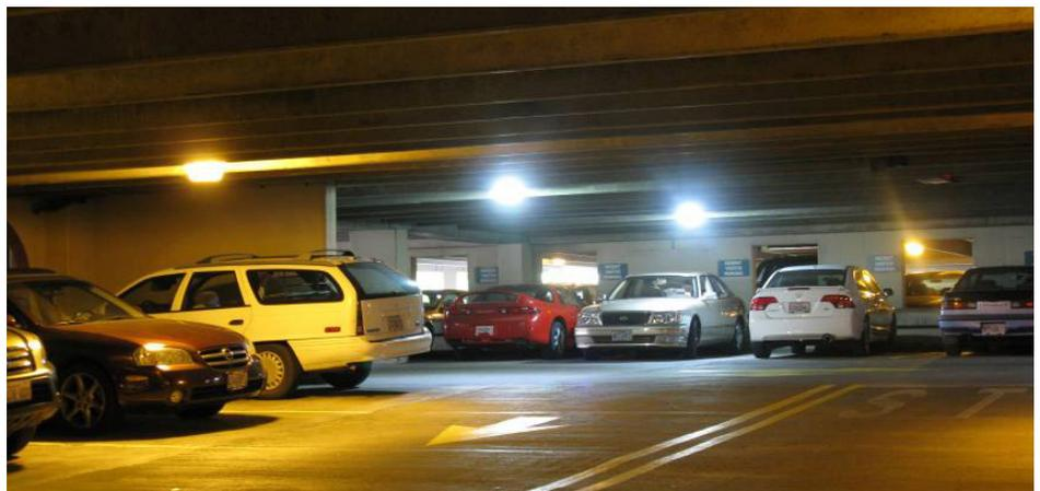
This comparison of LED and HPS lighting in another parking garage demonstration project conducted by PNNL shows how the brighter LED lighting dramatically improves color rendition and visibility.
