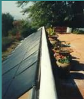
Solar Hot water
