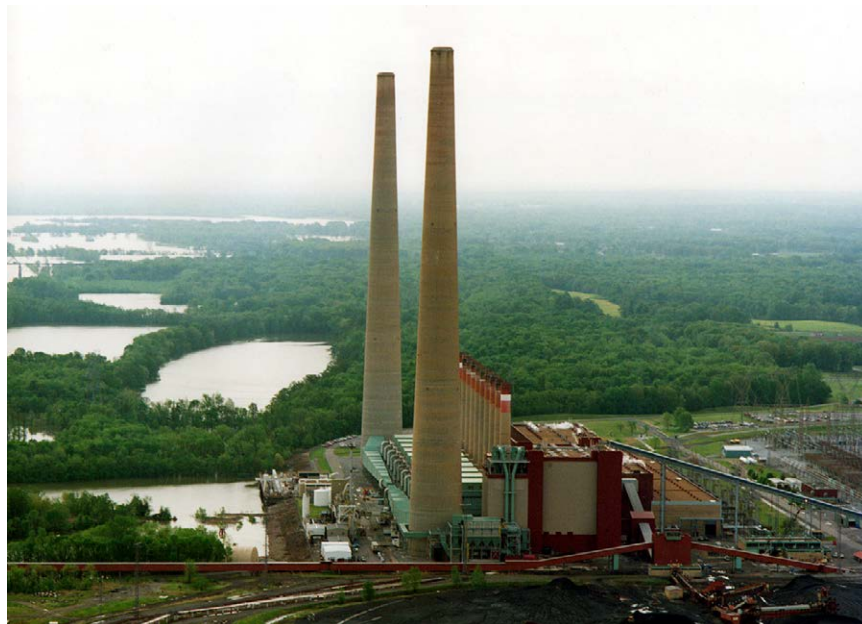
Figure 4-2. Aerial view of Shawnee Fossil Plant.
