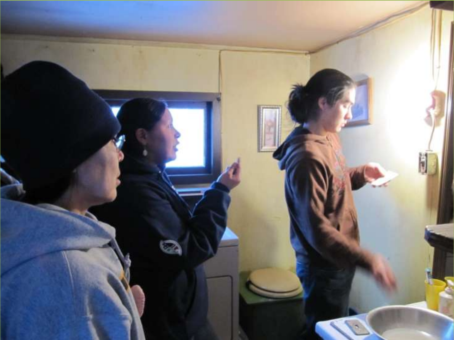
Placing insulation pads behind light switch plates and electrical outlets
