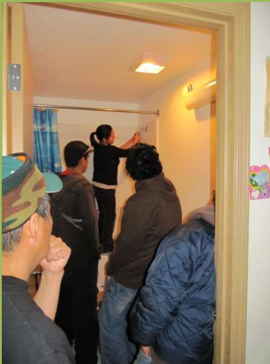
Installing low-flow shower-head
