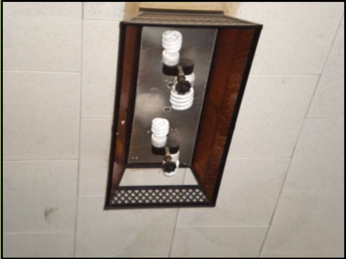
Replacing Incandescent with CFL bulbs
