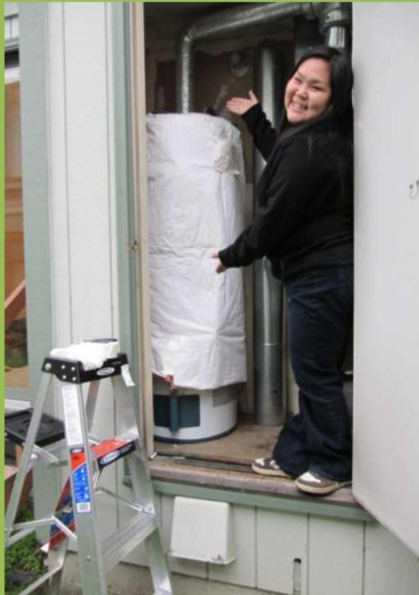
Wrapping hot water heater
