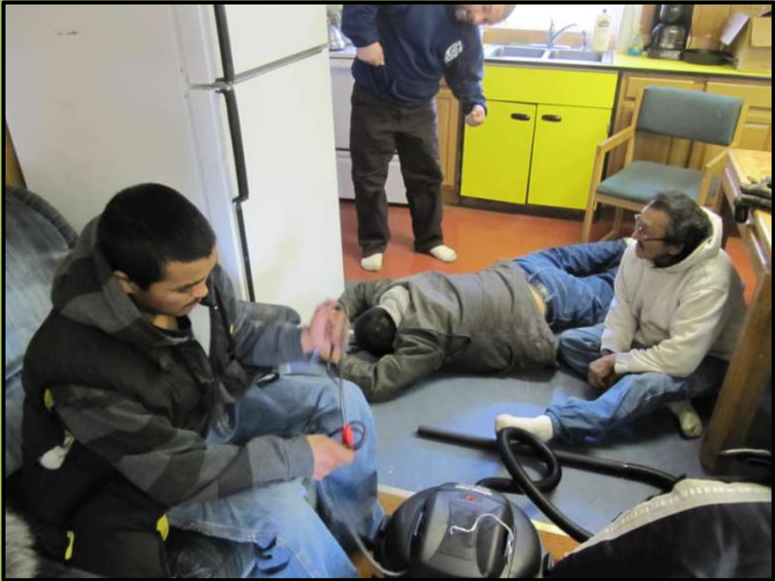
Cleaning refrigerator coils
