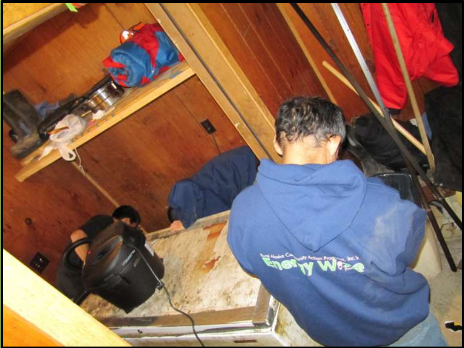
Cleaning freezer coils
