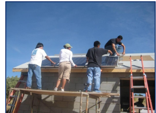
2008 Interns' participated in PV installation & training workshop (AZ-Hopi)
