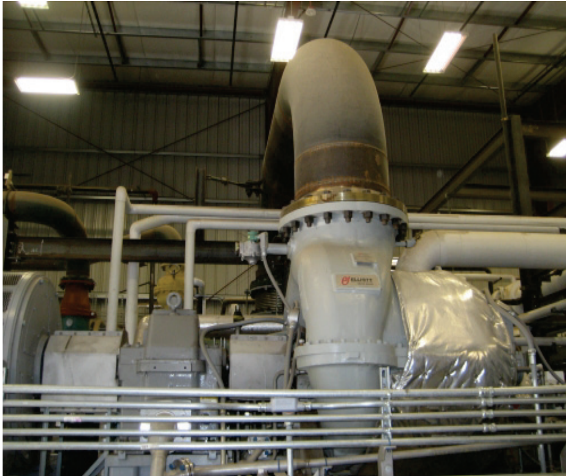
Carson Correctional Center Steam Generator
