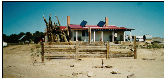
Solar Installations at Pueblo of Laguna's Majors Ranch
