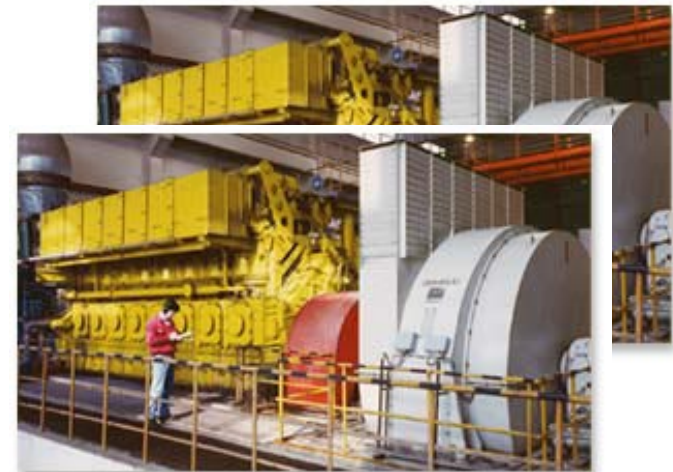
+ 2 570 kW Caterpillar Gas Generators
