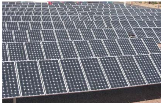
4 MW Single Axis Tracking System
