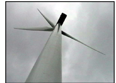
Turbine Installed at Rosebud Sioux Reservation in South Dakota
