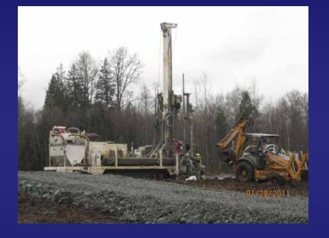
Drilling for one of 120 wells that are part of the geothermal heat pump for the new tribal administrative building – each well is approximately 350 feet deep.
