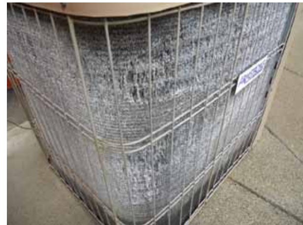
Typical outdoor condenser unit condition. Note damage to heat exchanger fins.
