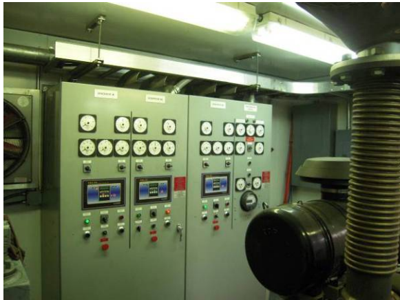
Power Plant Switch Gear - Overview
