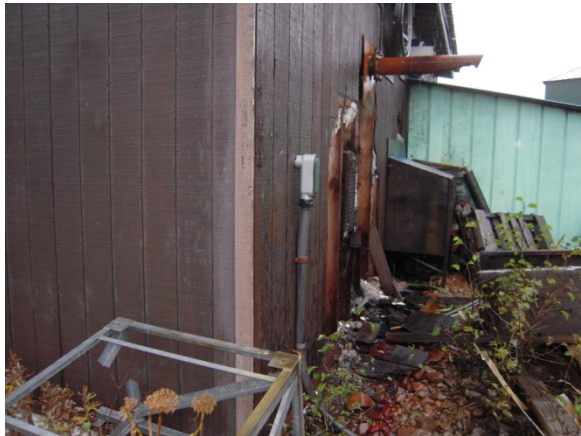
Old Power Plant – distribution service from new power plant
