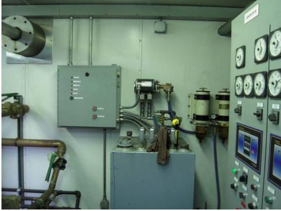
Power Plant Day Tank and Controls
