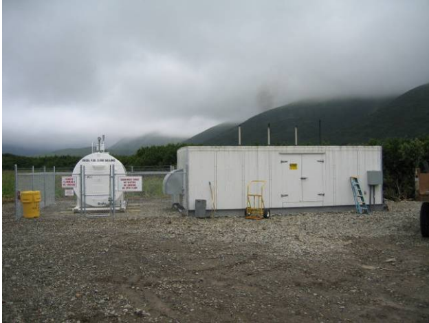
False Pass Power Plant with 5,000 gal. fuel tank.
