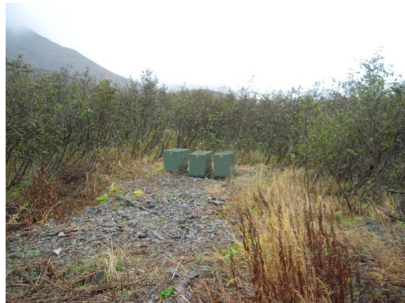
Distribution Transformers – Three phase from Old Power Plant feeders
