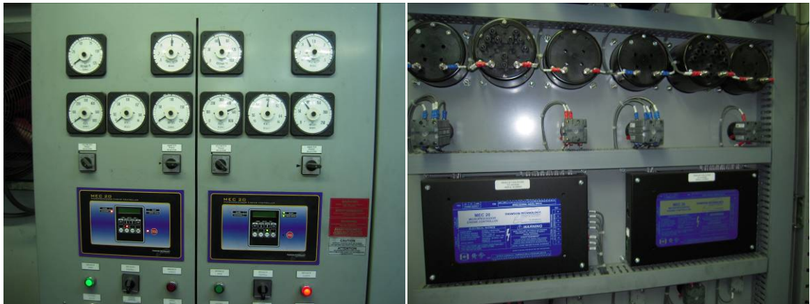
Power Plant Gen-Set Switch Gear – Close up
