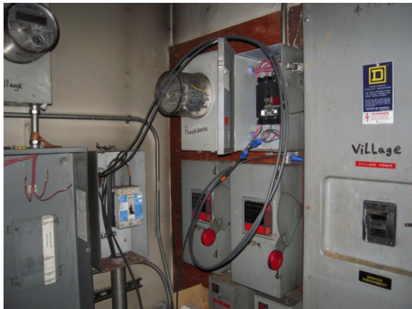
Old Power Plant – Village feeder and metering
