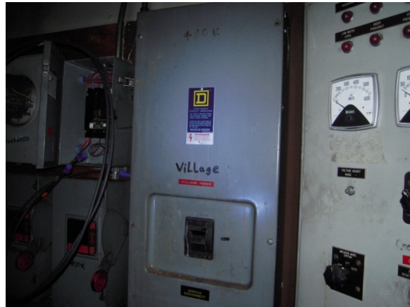
Old Power Plant – Village Feeder Switch
