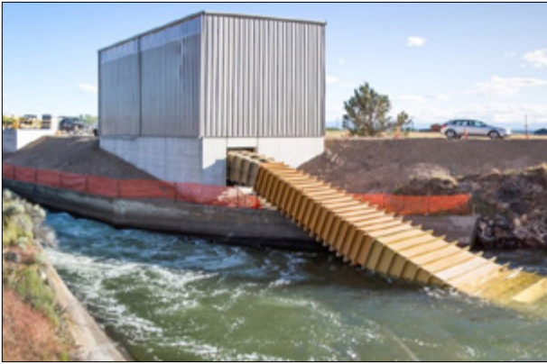
Natel Energy's Schneider Linear hydroEngine generates predictable, renewable energy for a previously unpowered, irrigation canal.
