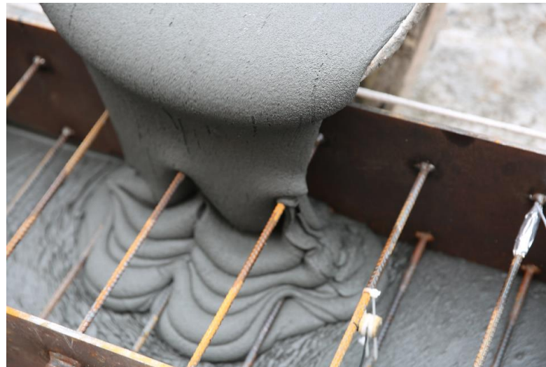
Casting of S-UHPC beam
