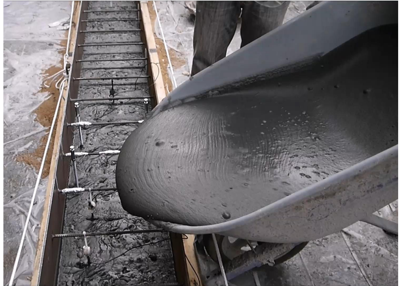
During casting of Steel-plate UHPC beam, good flowability demonstrated without vibration
