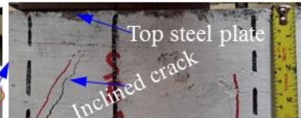
(b) Crack close top steel plate
