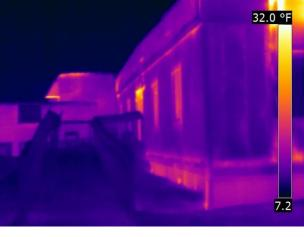
doors are in good condition but lack proper sealing into door frame because of worn weather stripping and/or improper fit.
