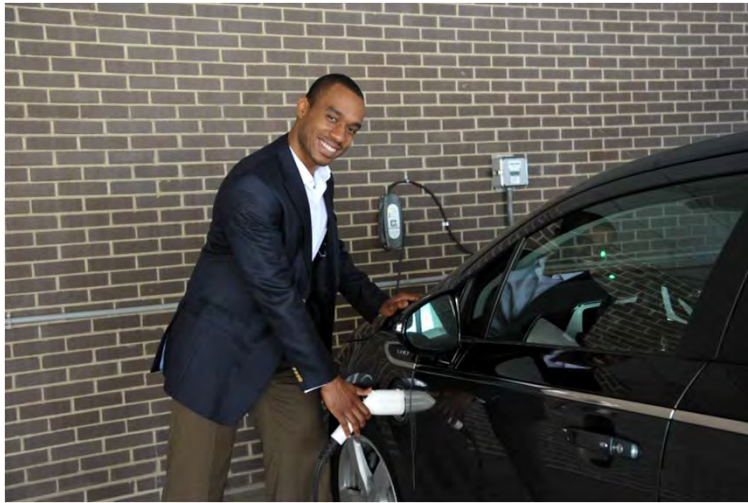
Employee charging stations installed at the Authority's White Plains office
