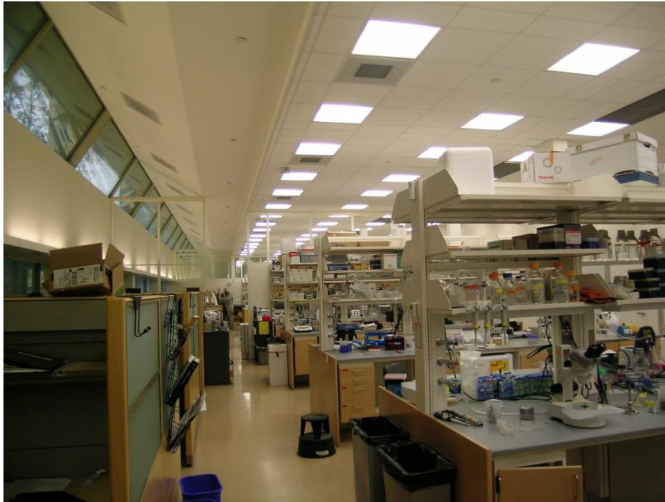
Figure 3: Laboratory space in the Carl Icahn Laboratory, showing the recessed 2x2 fluorescent troffers and the linear fluorescent cove fixtures along the perimeter.
