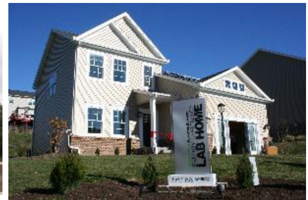
Two Story Basement
