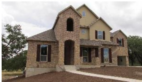
Two Story Slab
