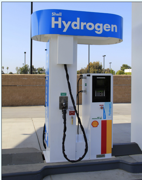
The first hydrogen fueling station in America, supplied directly from an active industrial hydrogen pipeline, provides hydrogen for demonstration fuel cell vehicle fleets in the Los Angeles area. The station is a collaborative effort among the Energy Department, Toyota, Air Products, Shell, and South Coast Air Quality Management District (SCAQMD). Source: NREL/Michael Penev
