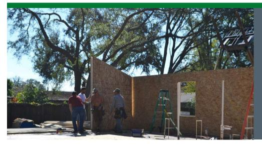
The home was constructed with 6.5-inchthick (R-26) SIP wall panels and 8.25-inch (R-34) roof panels. The panel's inner core of foam provides a nearly continuous thermal layer around the home. The solid panels with their interlocking glued joints also form a solid air barrier around the home.
