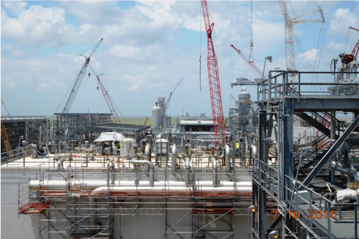
Train 1 – Pipe alignment on top of Methane Cold Box
