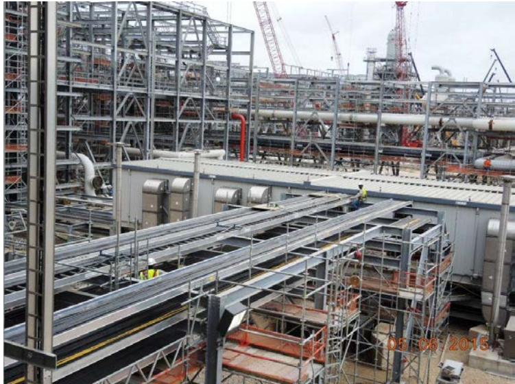
Train 1 Compressor Substation – Pulling Cable
