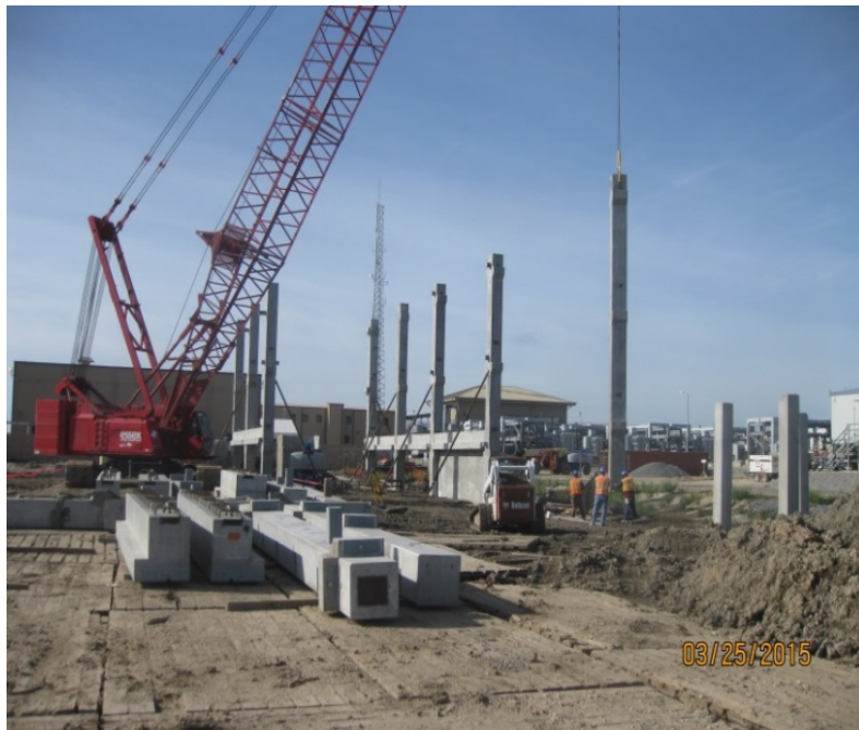
Crane placing pre-cast columns for the maintenance shop.
