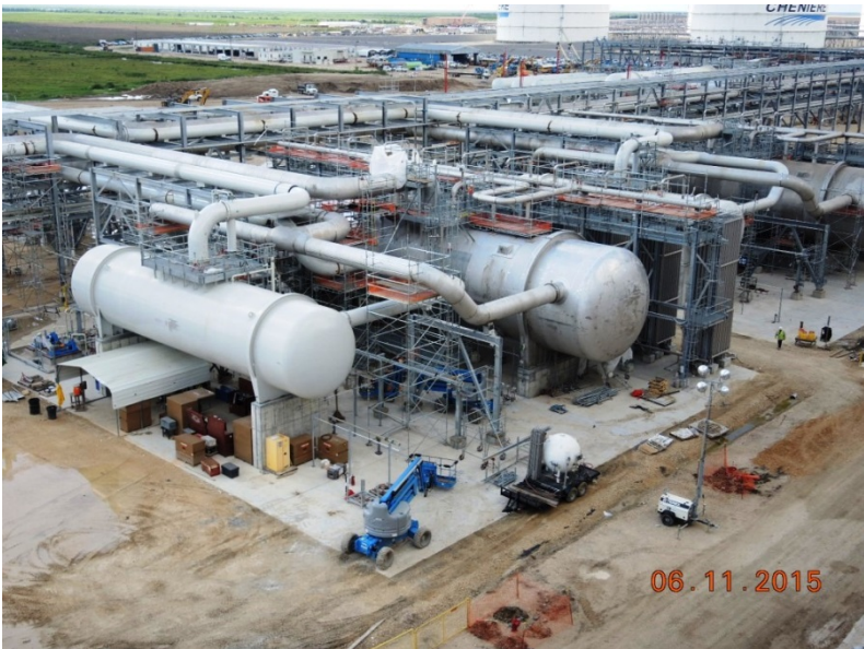
Stage 2 OSBL Flare Knockout Area – Installing Pipe
