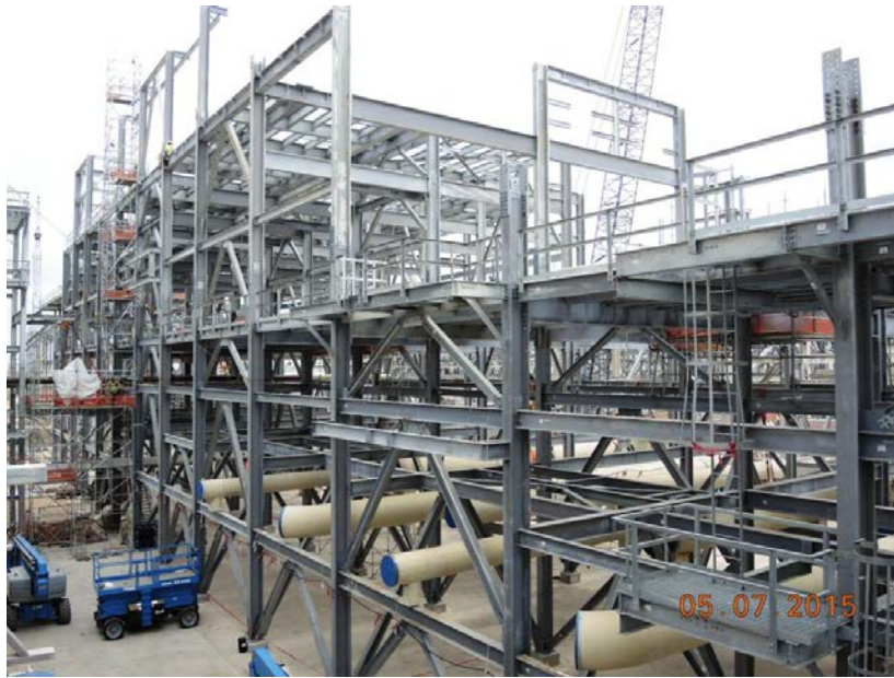
Train 4 Cryorack Air Coolers and Piperack Area – Installing Upper Steel
