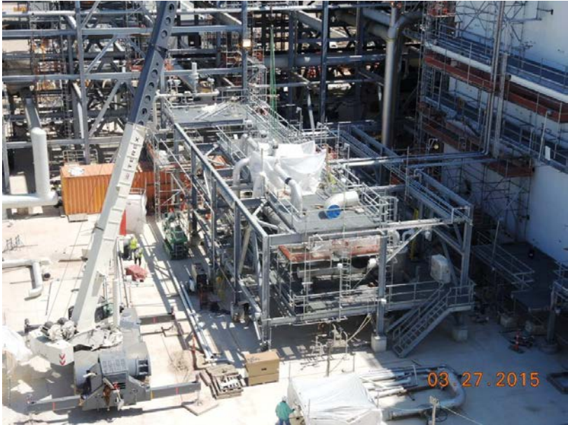
Train 2 Methane Cold Box – Installing Pipe
