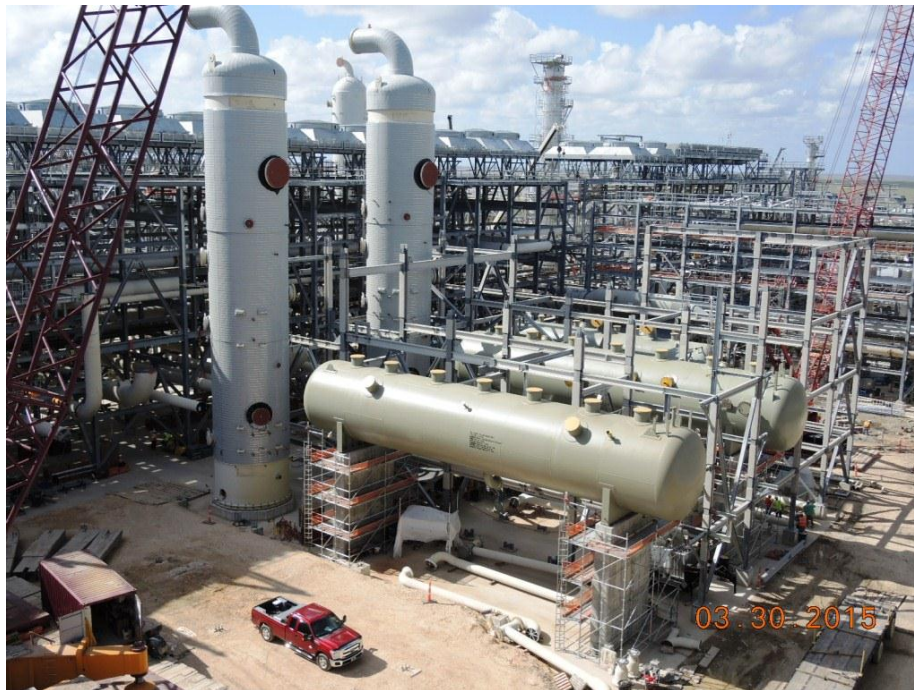
Stage 2 Propane Refrigeration Feed Chillers, Suction Drums and Cryorack Coolers
