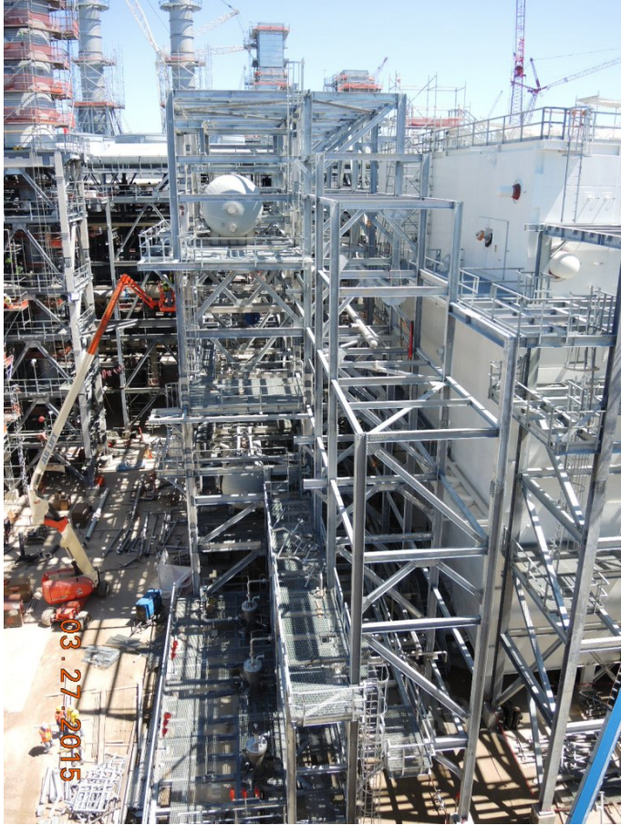
Train 2 Ethylene Cold Box – Installing Steel
