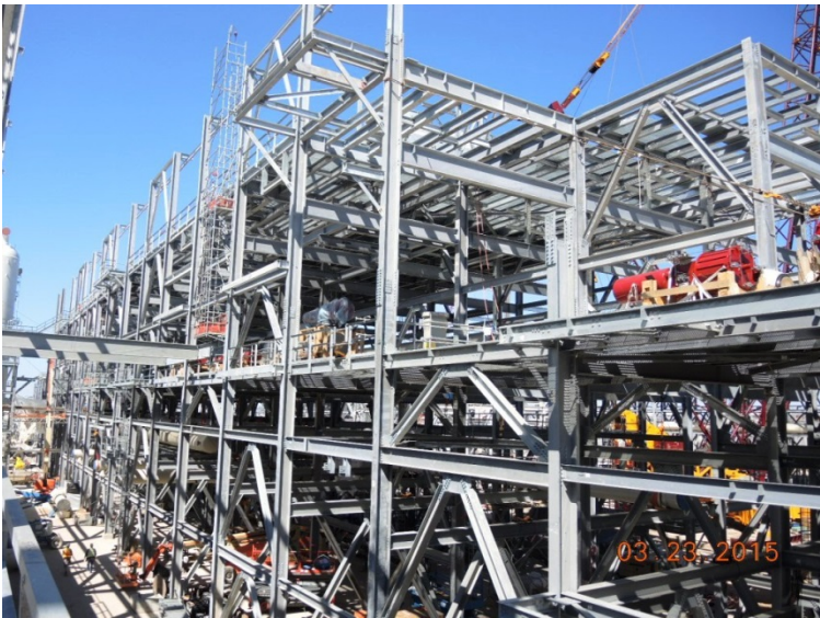
Train 3 Cryorack – Erecting Upper Steel Package
