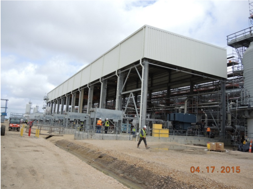
Stage 1 OSBL BOG Compressor Area
