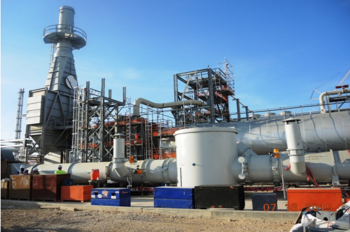
Stage 2 OSBL Thermal Oxidizer Area – Piping
