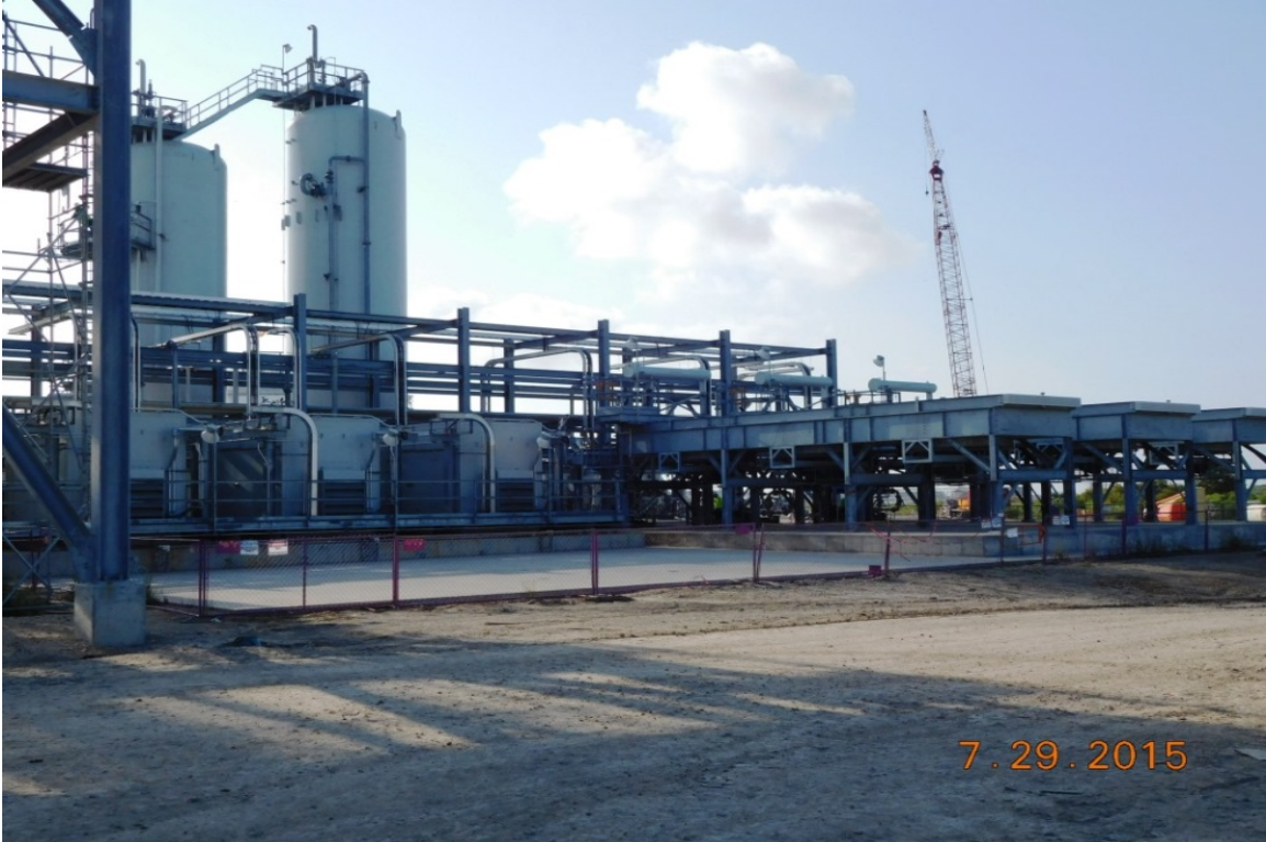
Stage 1 OSBL Instrument Plant Air Area – Turnover to Startup
