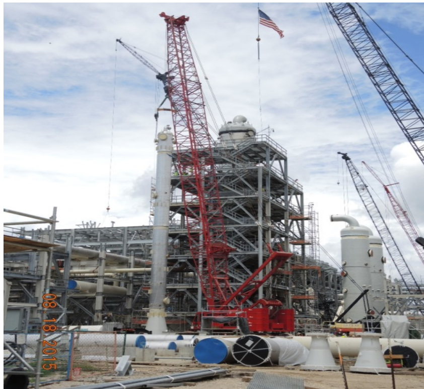
Train 4 Heavies Removal Area – Setting Debutanizer
