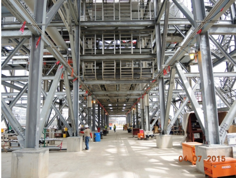
Train 3 Propane Condenser Piperack – Installing Cable Tray
