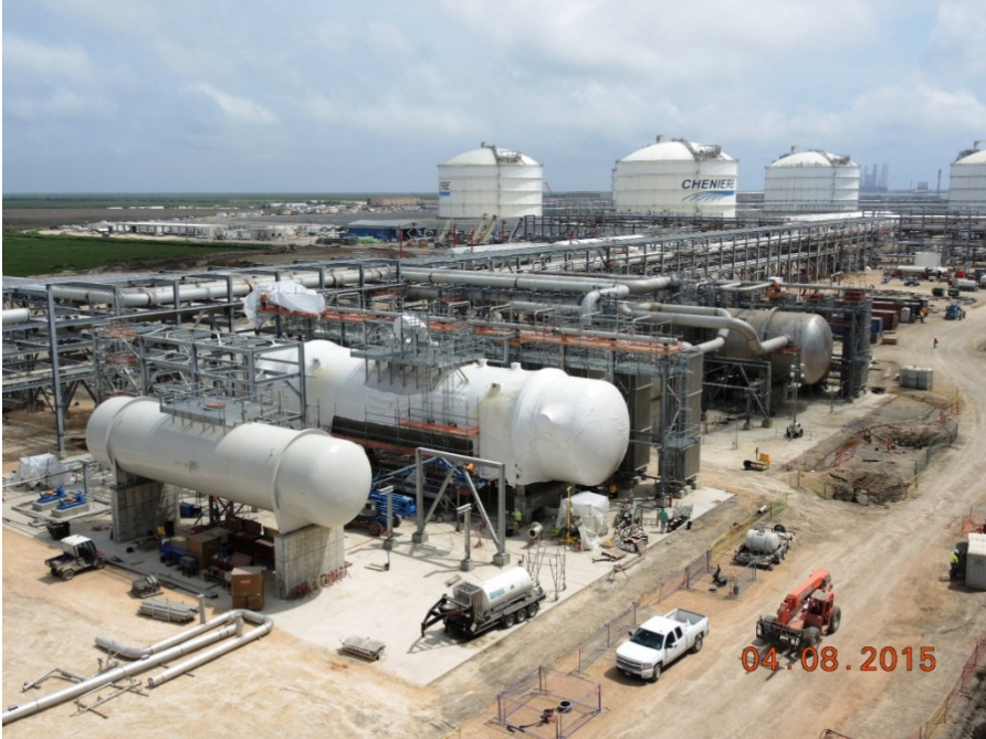
OSBL 2 Flare Knockout Drums Area – Installing Platforms
