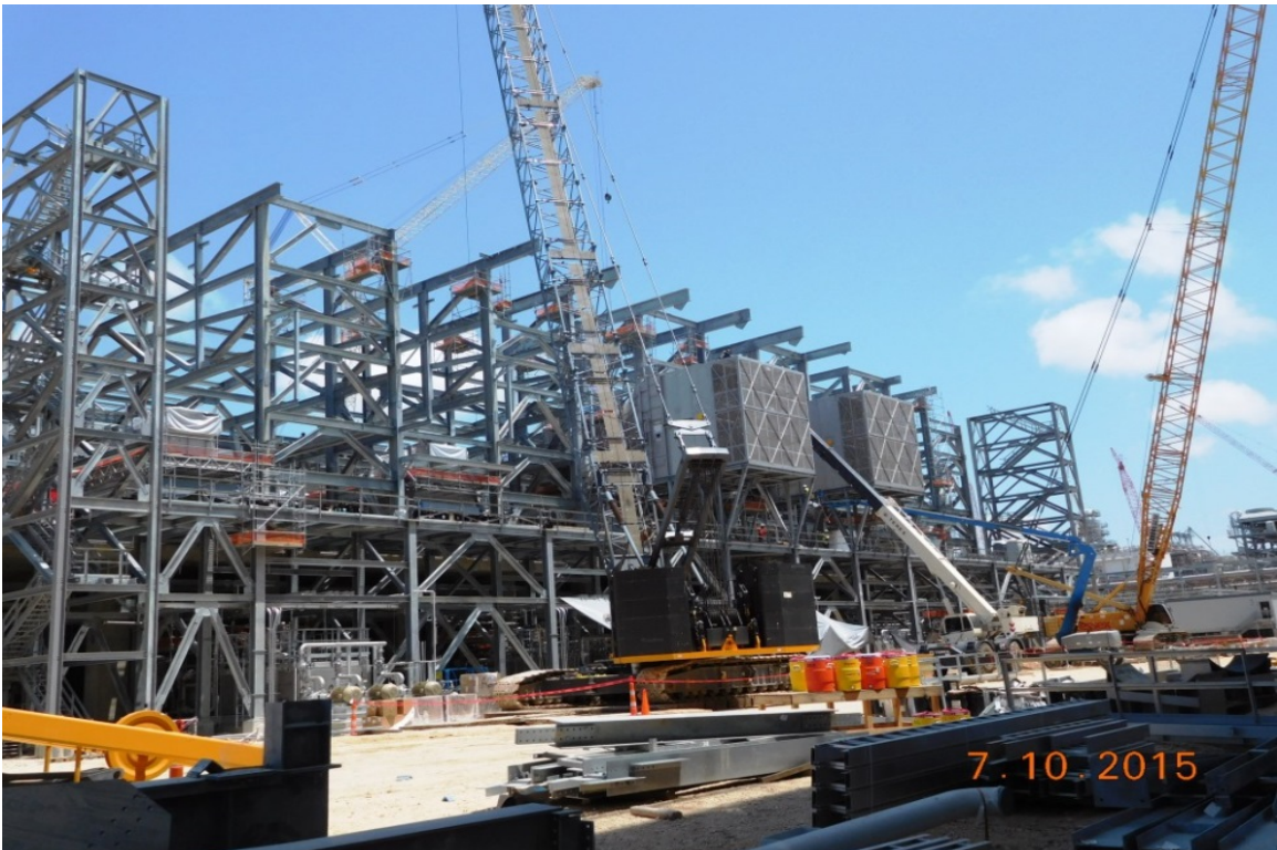
Train 3 Compressor Area – Setting Filter House
