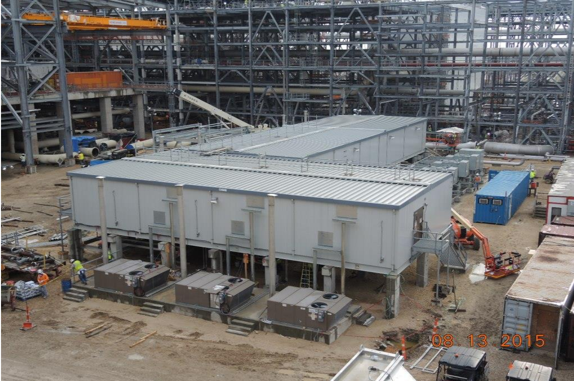
Train 3 Compressor Substation Building
