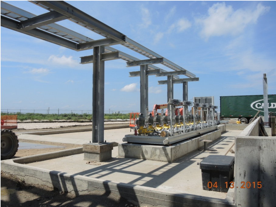
OSBL 2 Utilities Waste Water & Solvent Area – Scavenge Metering Pump Skid
