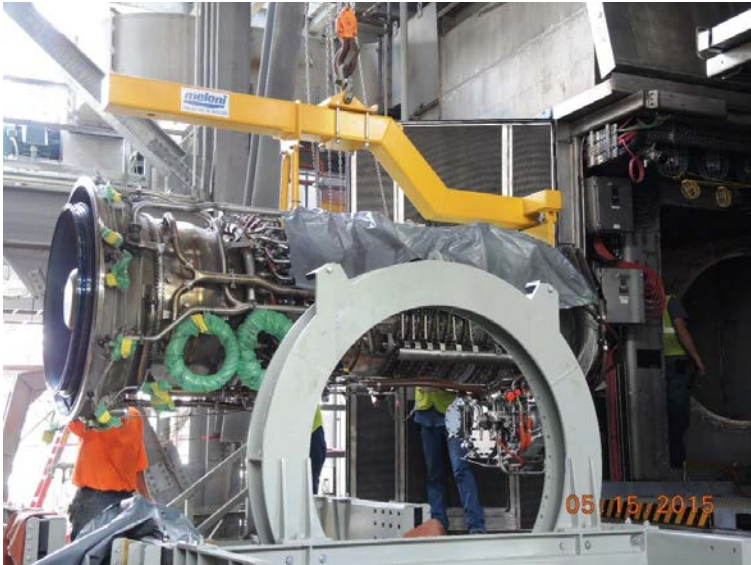
Train 1 Compressor Area – Installing Gas Generator
