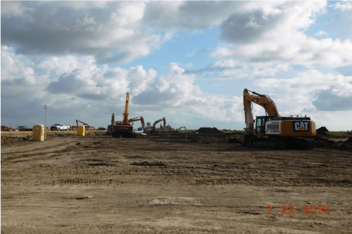
Stage 3 Soil Stabilization work in progress
