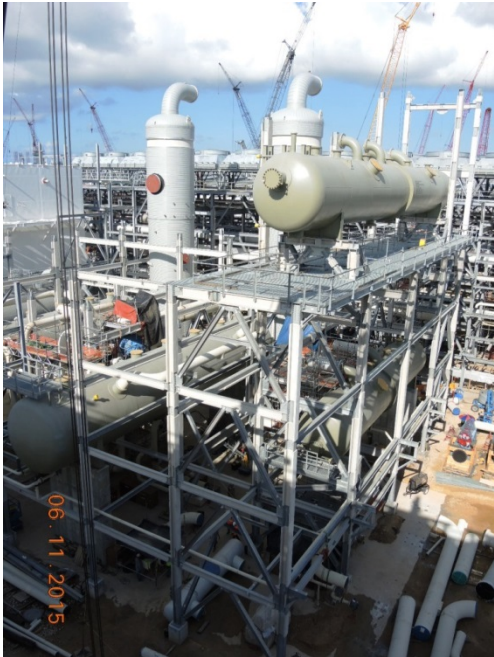
Train 3 Propane Refrigeration Area – Setting I.S. Propane-Methane & Ethylene Feed Chiller
