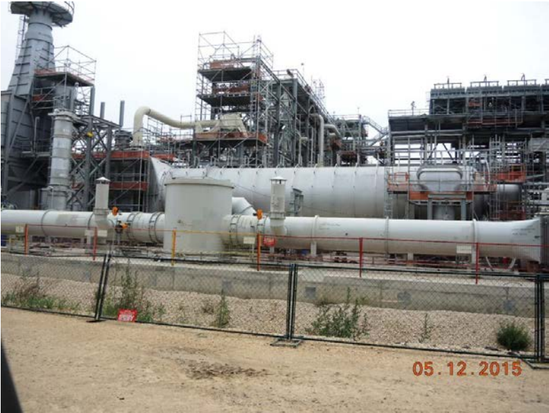
Train 2 Thermal Oxidizer Area
