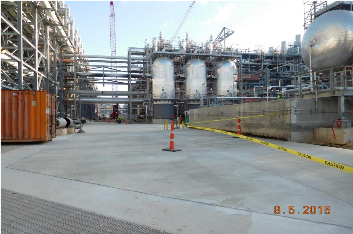
Train 2 Propane Condenser Area - Paving
