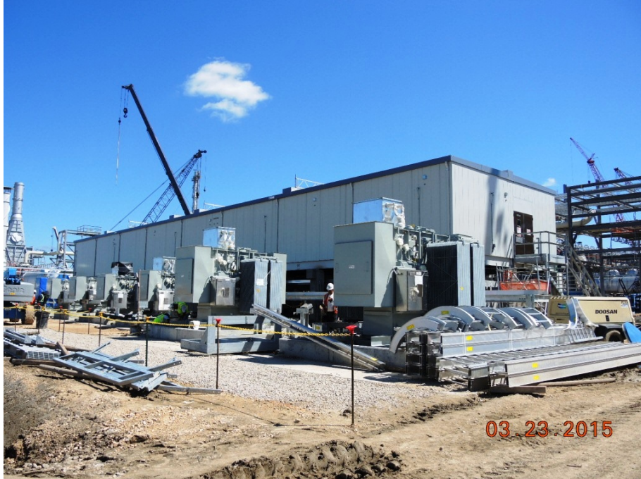
Stage 2 OSBL Utility Station Area – Transformers Installed
