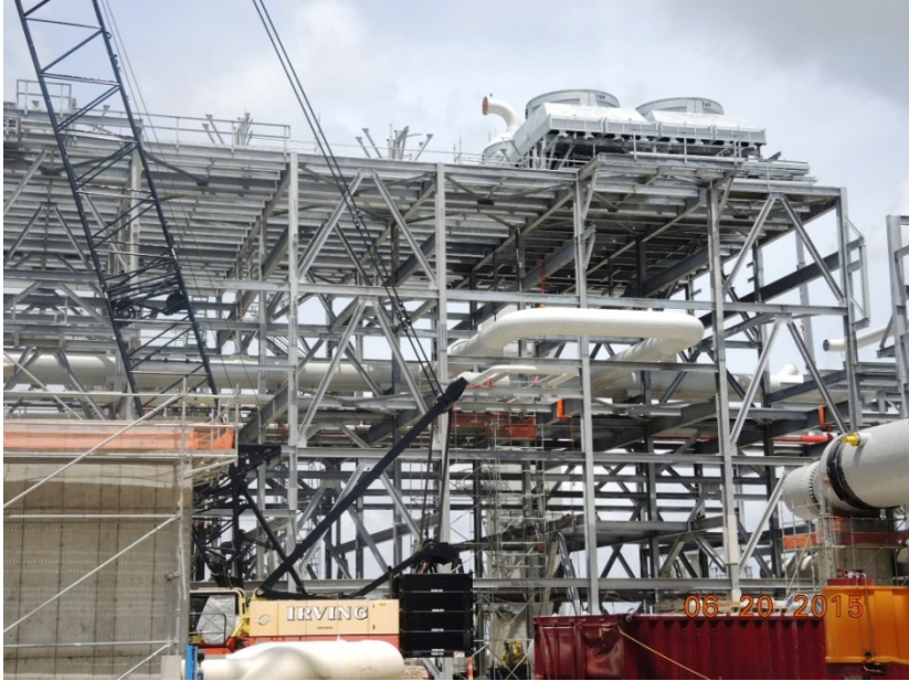
Train 4 Cryorack Air Coolers and Piperack Area – Setting Absorber Overhead Gas Coolers
