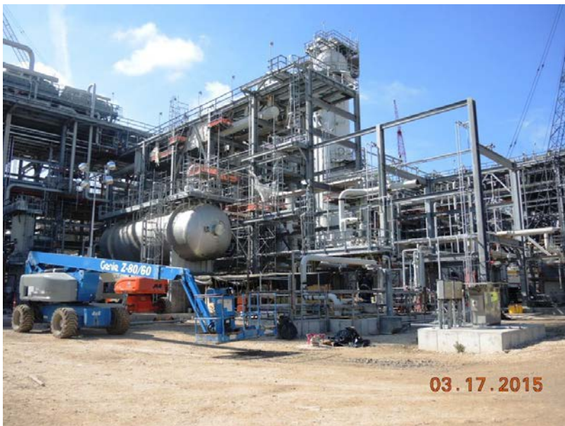
Train 1 Amine Regen and Acid Gas Removal – Installing Pipe
