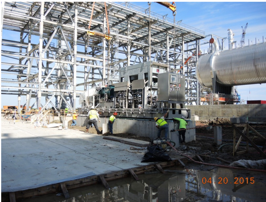
Train 4 Dehydration & Mercury Removal Area – Setting Regen Gas Compressor
