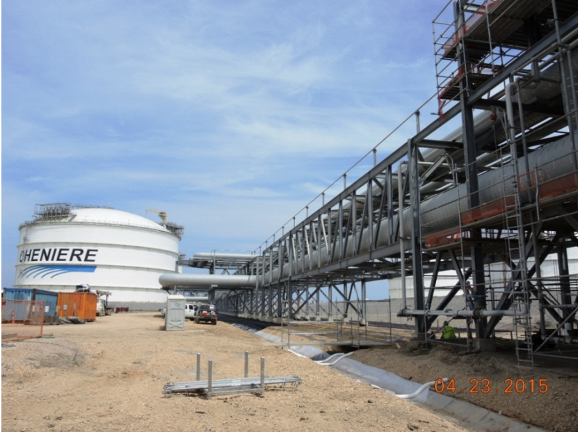
Train 1 & 2 OSBL Utilities Pipe Rack – Pipe Insulation
