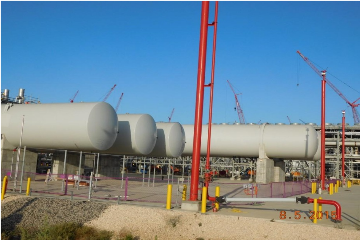
Stage 1 OSBL Refrigerant Storage Area – Turnover to Startup
