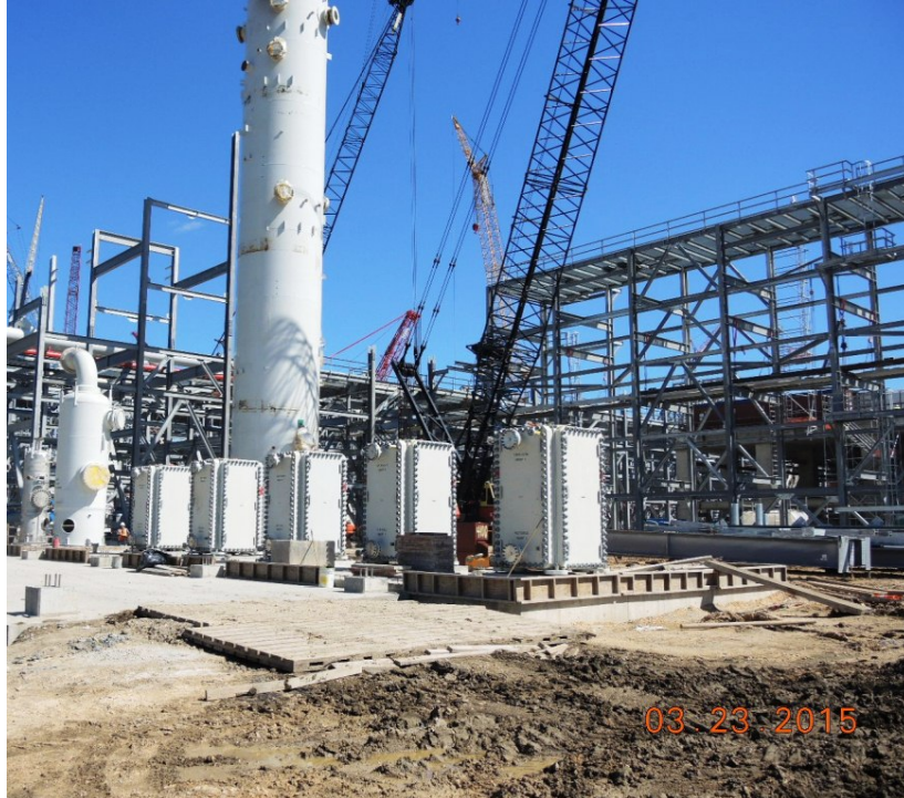
Train 4 Amine Regen/Acid Gas Removal Area – Lean Rich Solvent Heat Exchangers Installed
