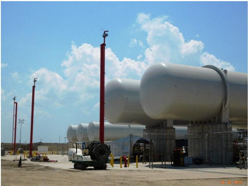
Stage 1 OSBL Refrigerant Storage Area – Firewater Monitors Installed
