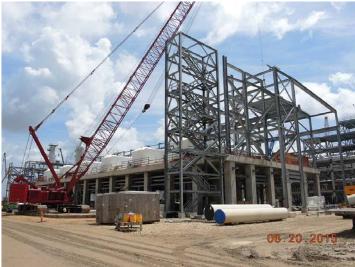
Train 4 Compressor Area – Setting Steel Above the Table Top
