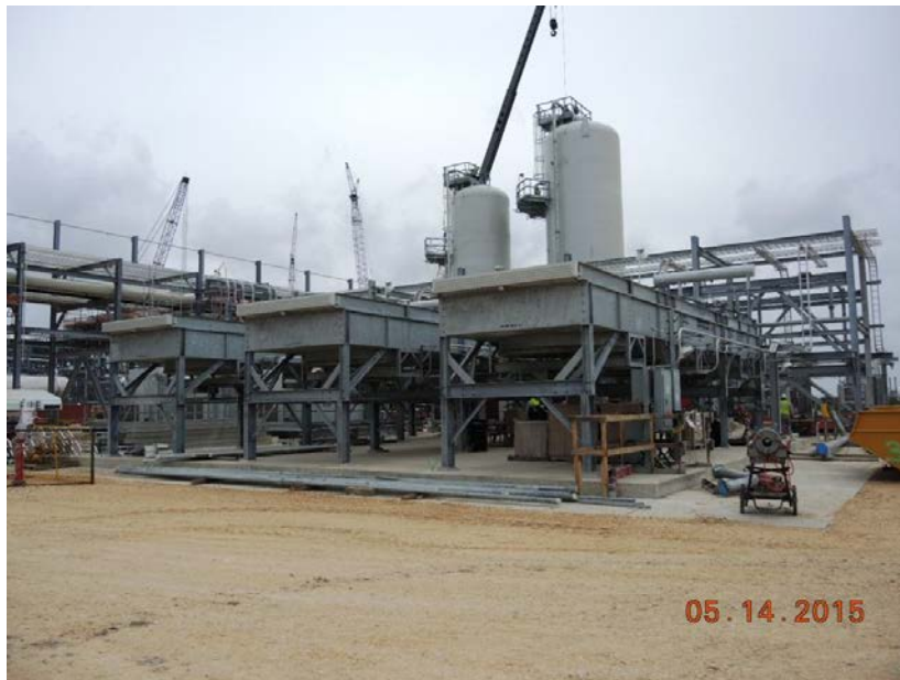
Stage 2 OSBL Instrumentation Plant Air Area– Cooling Water Exchanger Skid
