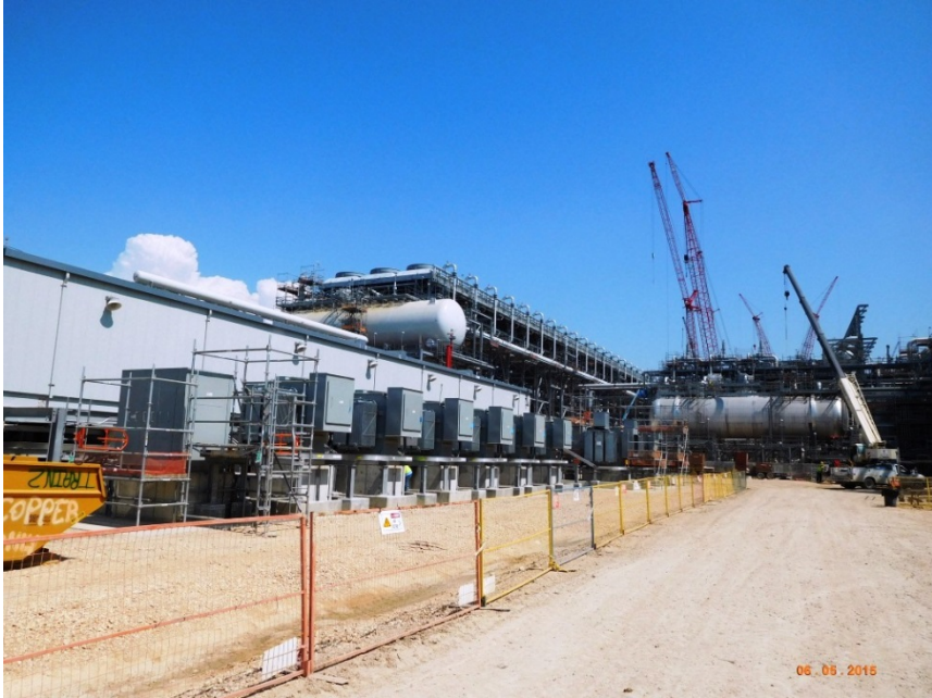
Train 2 Propane Substation Energized
