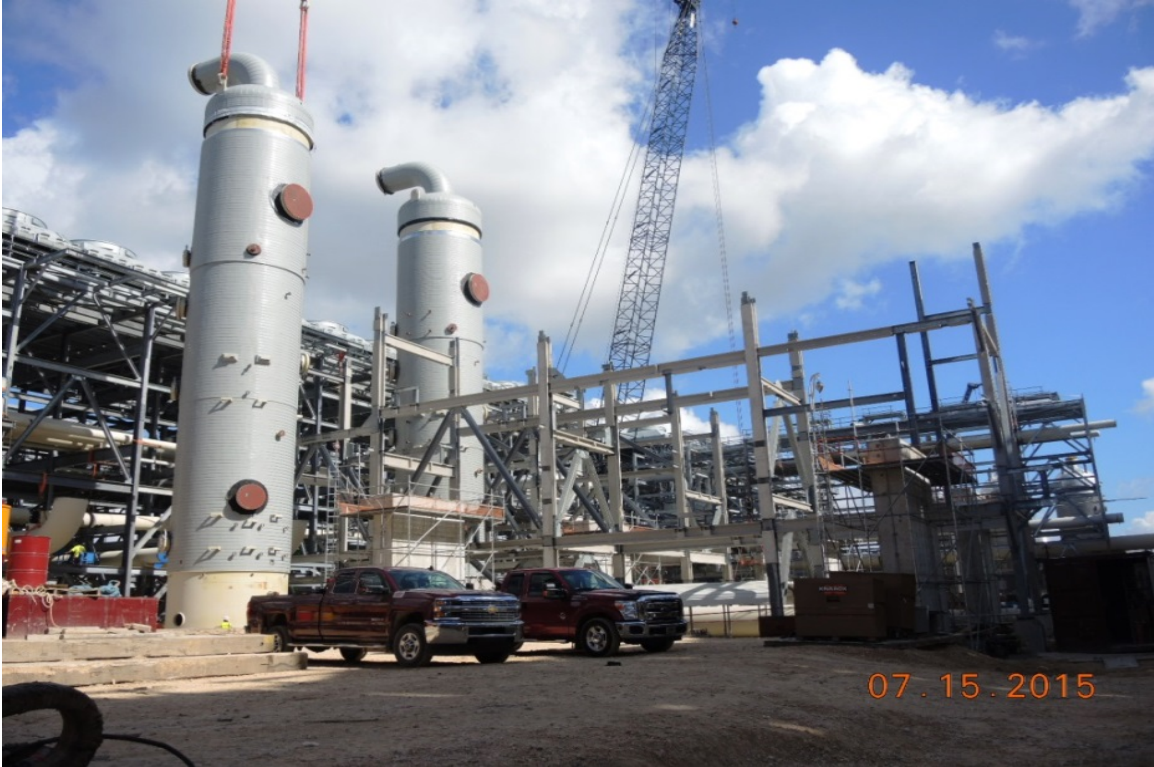
Train 4 Propane Refrigeration Area – Setting Low Stage Propane Suction Drums
