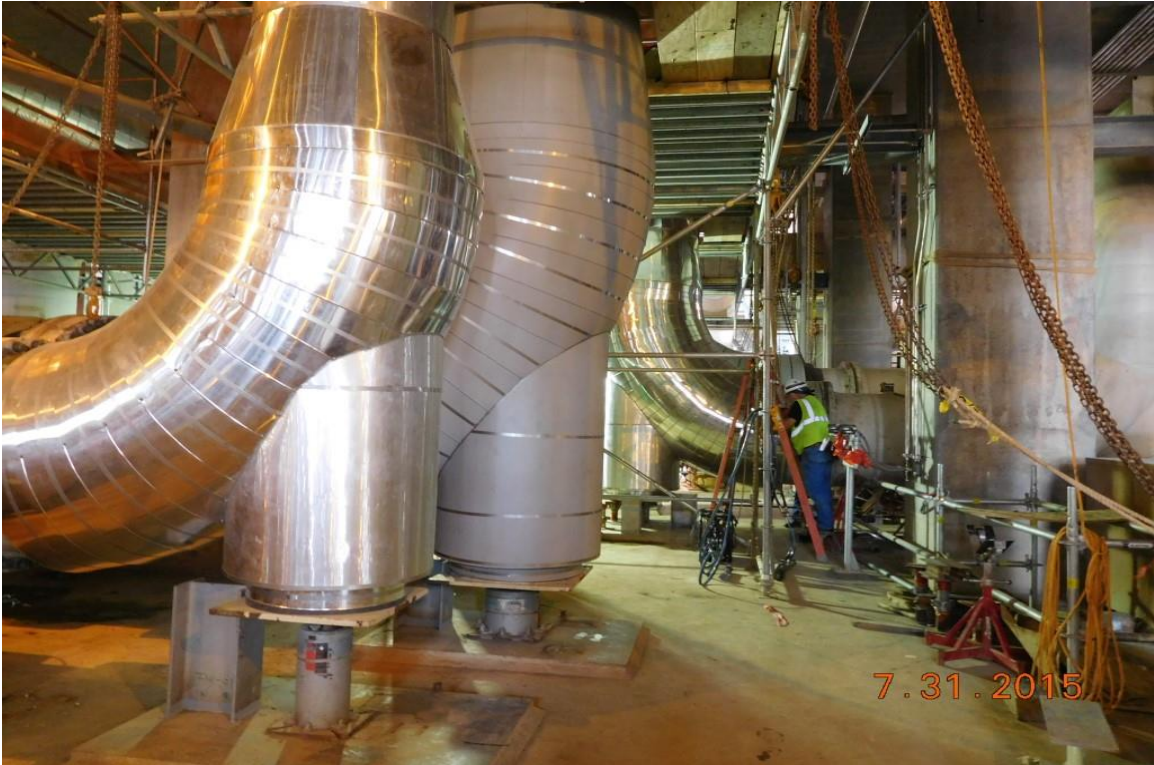
Train 1 – Pipe insulation under the Compressor Box
