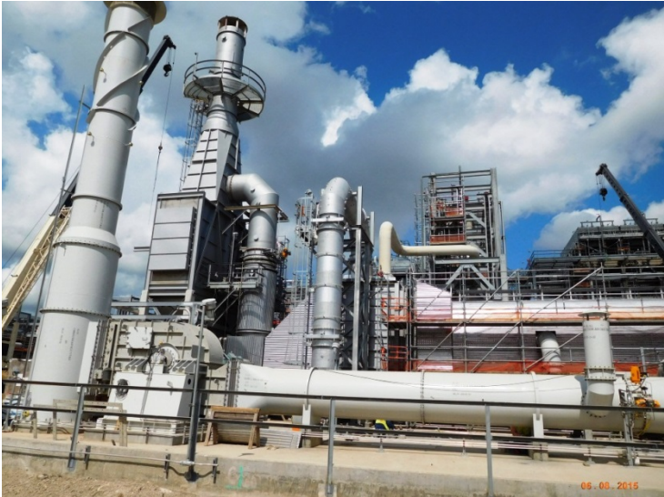
Train 1 Thermal Oxidizer – Installing Insulation
