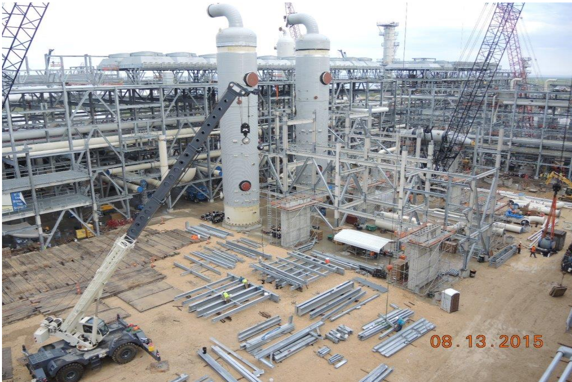
Train 4 Propane Refrigeration Area – Erecting Steel
