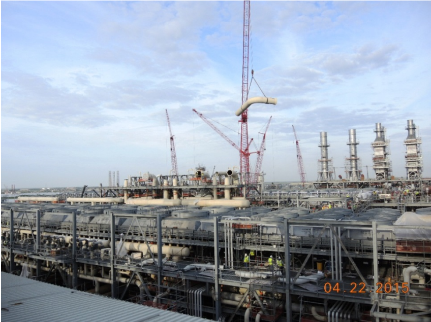
Train 1 Propane Refrigeration Area – Installing Pipe
