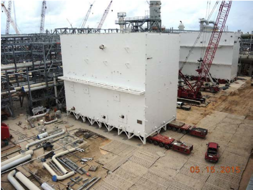
Train 3 – Setting Methane Cold Box
