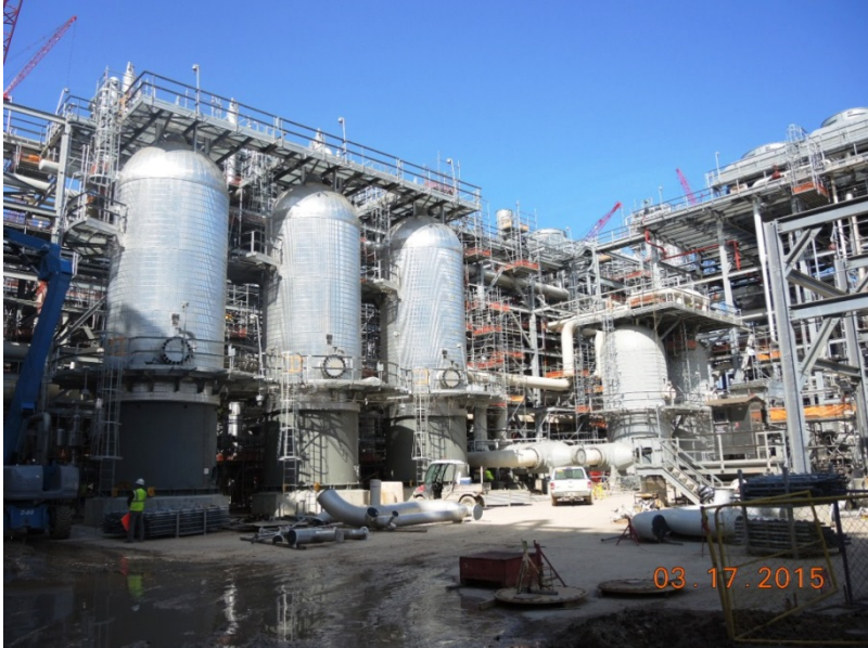
Train 1 Molecular Sieve Dehydrators and Mercury Removal Beds
