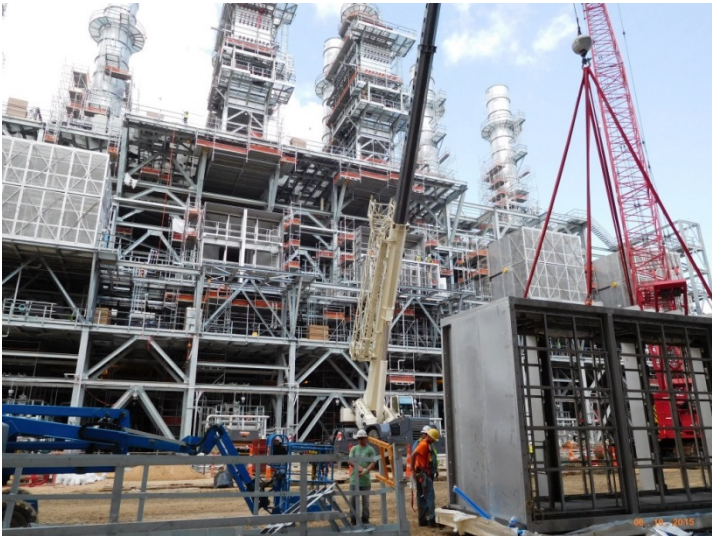
Train 2 Compressor Area – Installation of Filter Houses
