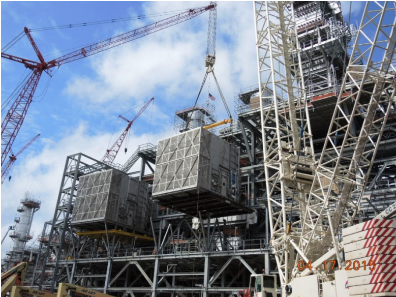
Train 2 Compressor Area – Installing Propane Filter Houses
