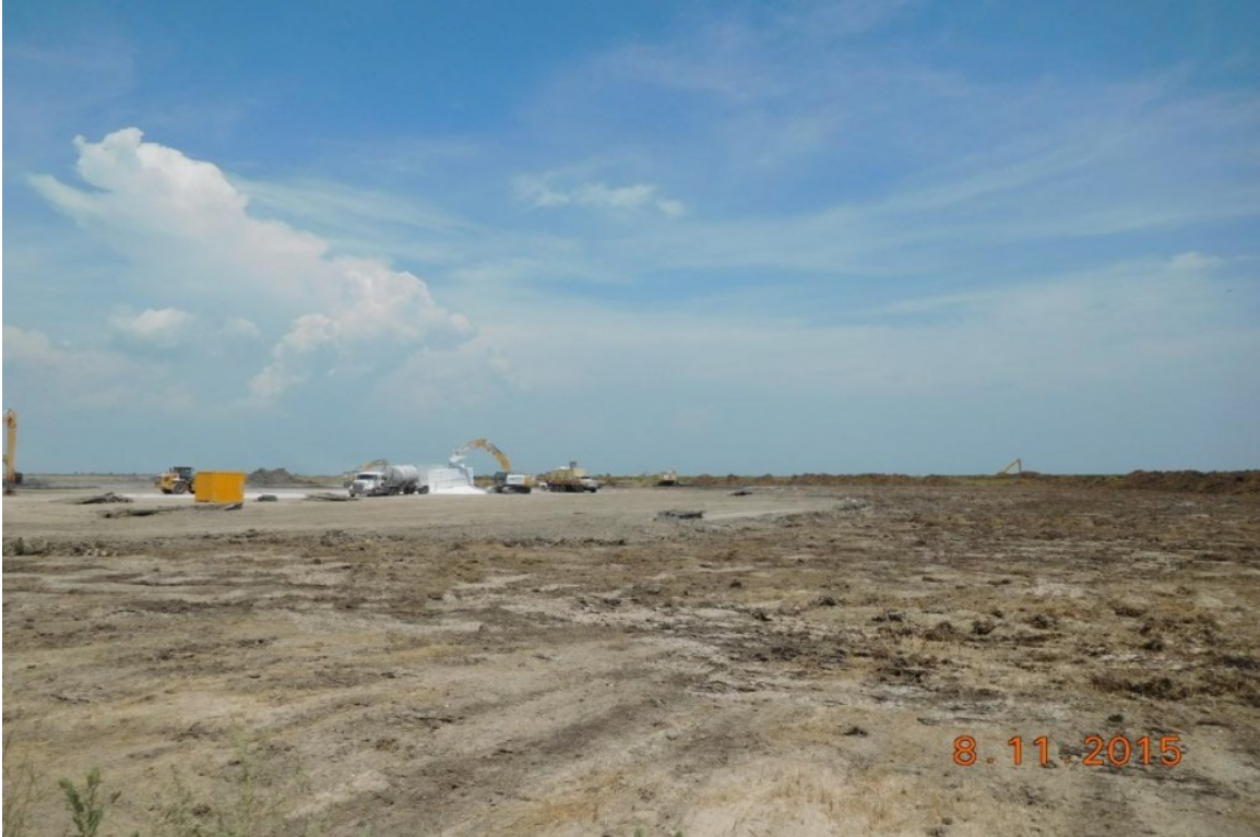
Stage 3 Soil Stabilization
