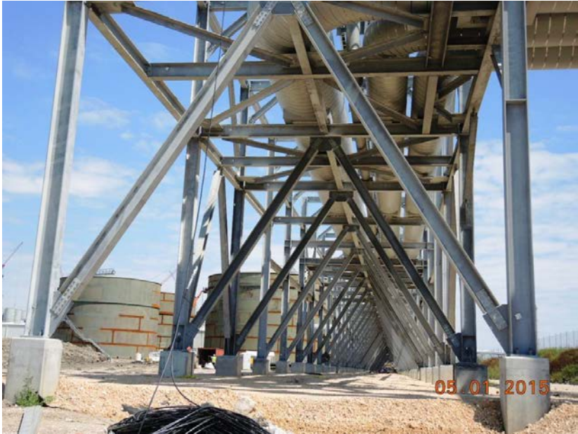
Stage 1 OSBL North/South Piperack – Pulling Cable
