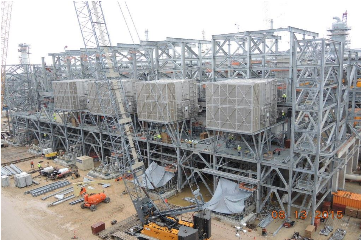
Train 3 Compressor Area – Setting Filter Houses
