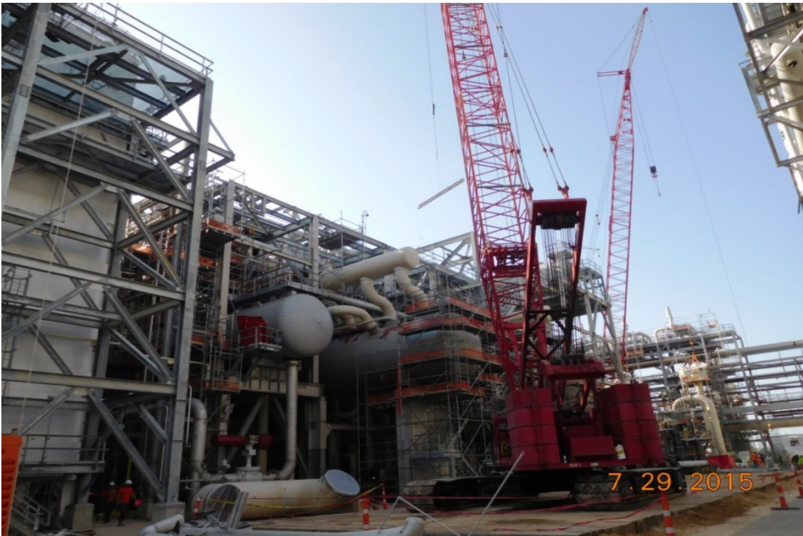
Train 2 Propane Refrigeration Area – Steel Installation
