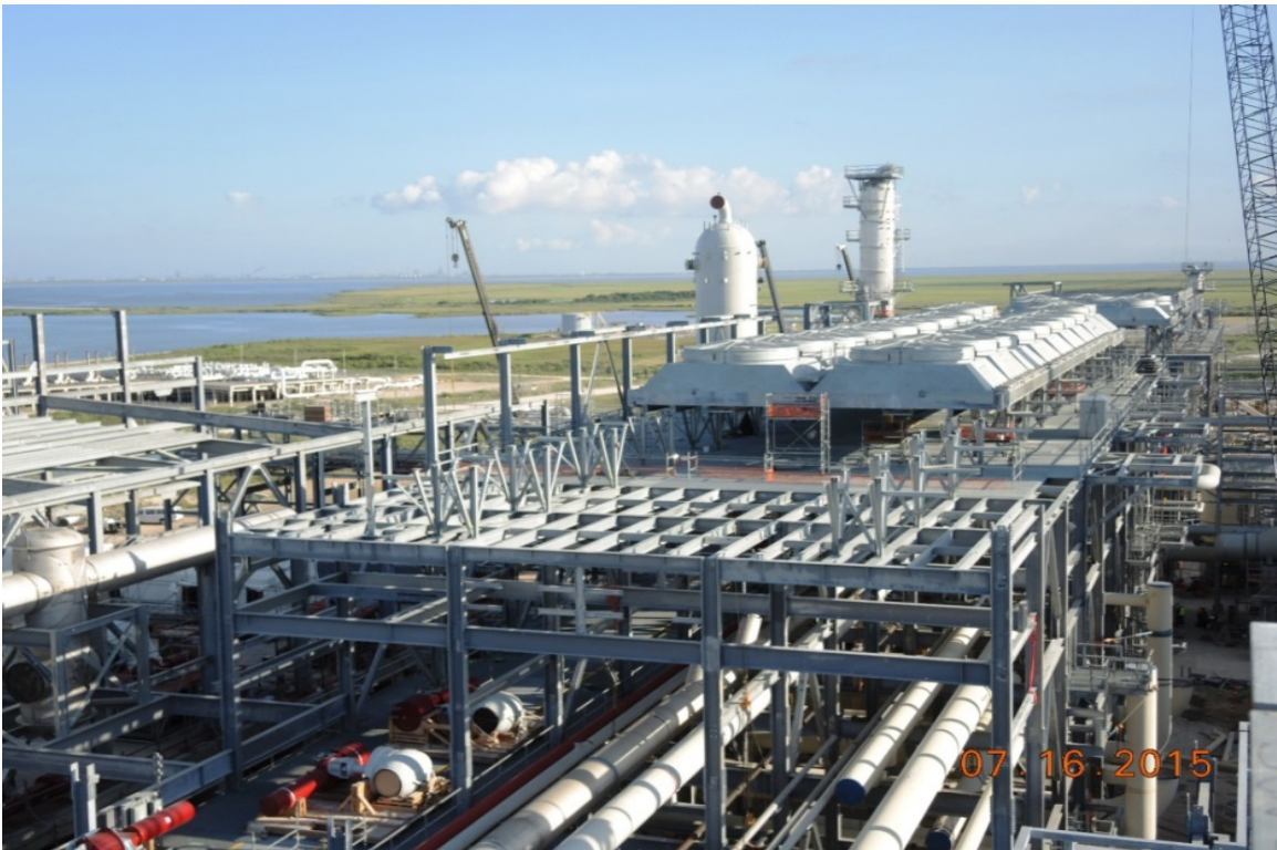
Train 4 Cryo Rack Area – Setting Coolers
