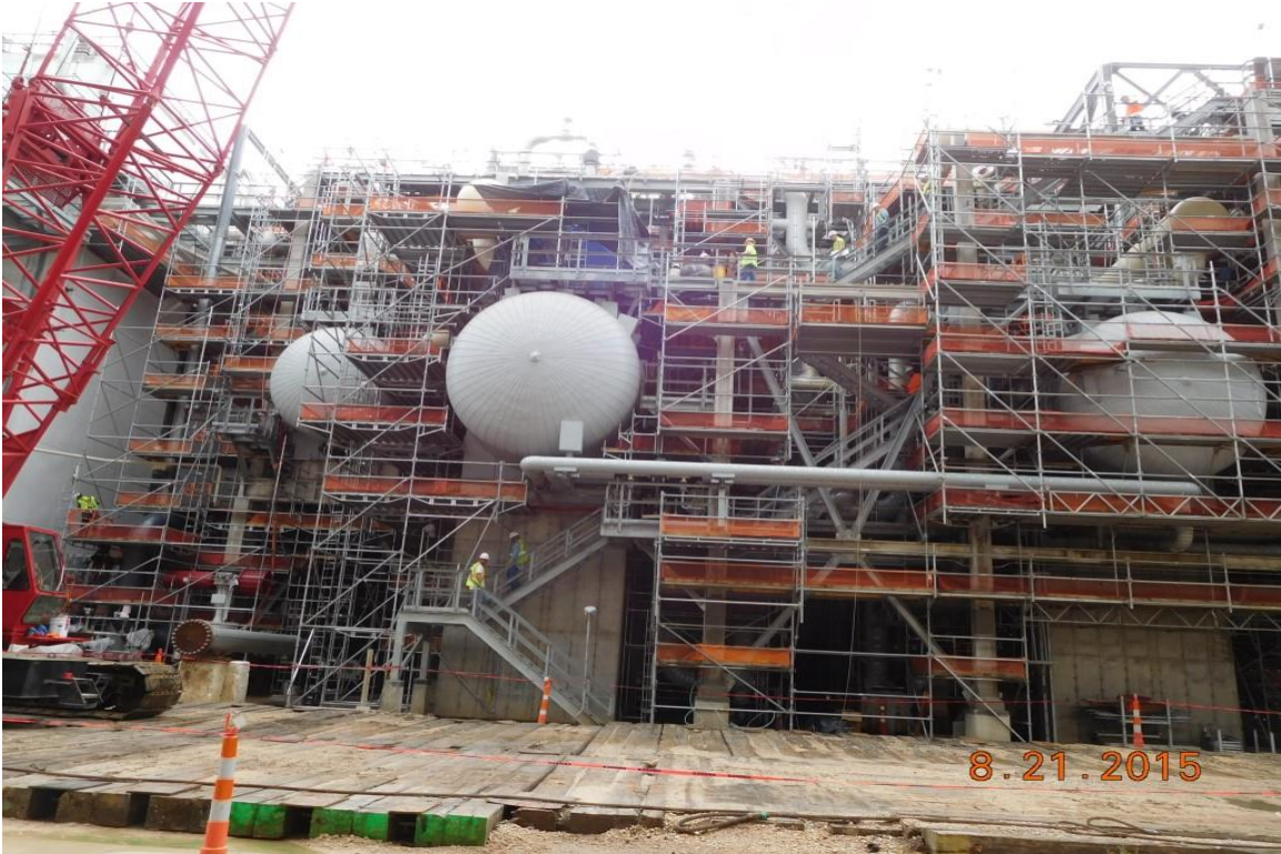
Train 2 Propane Refrigeration Area - Fireproofing
