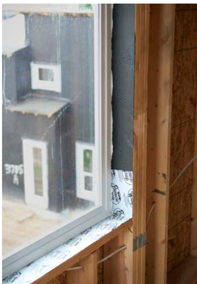
The black asphalt emulsion coating provides a seamless weather-resistant barrier on the exterior of the homes and windows.
