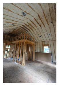
The home's wall framing is extensively air sealed, then the walls and attic roof are filled with open-cell spray foam for a quiet, thermal blanket.
