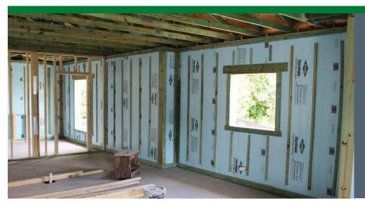
A continuous layer of rigid EPS foam insulation slows the transfer of heat through the walls. Borate-treated framing is more resistant to bugs and mold than untreated wood. The hurricane straps visible here, together with the roof's hip design, lack of soffit vents, and spray foam insulation, could help to keep the roof intact and in place in a hurricane.
