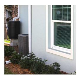
High-efficiency windows keep out unwanted solar heat gain, while gutters and downspouts direct rainwater away from the structure. Native, drought-tolerant plants helped the home meet the requirements of the Florida Green Building Coalition's Florida Green Home requirements, Florida Water Star, and the University of Florida's Florida Friendly Landscape program.
