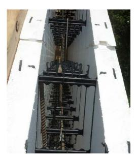
Insulated concrete form (ICF) blocks stack up to form hollow walls that are reinforced with steel and filled with concrete for a very sturdy wall that is resistant to wind, tornados, hurricanes, earthquakes, fire, and pests.
