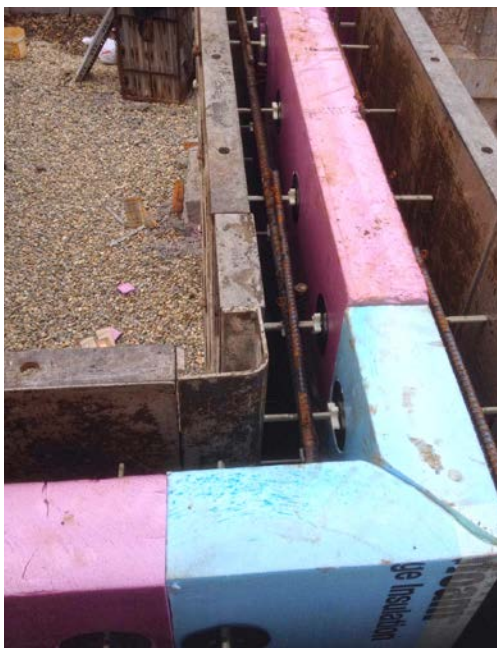
The 14-inch-thick foundation walls include a 4-inch XPS (R-20) rigid foam core, sandwiched between layers of concrete.
