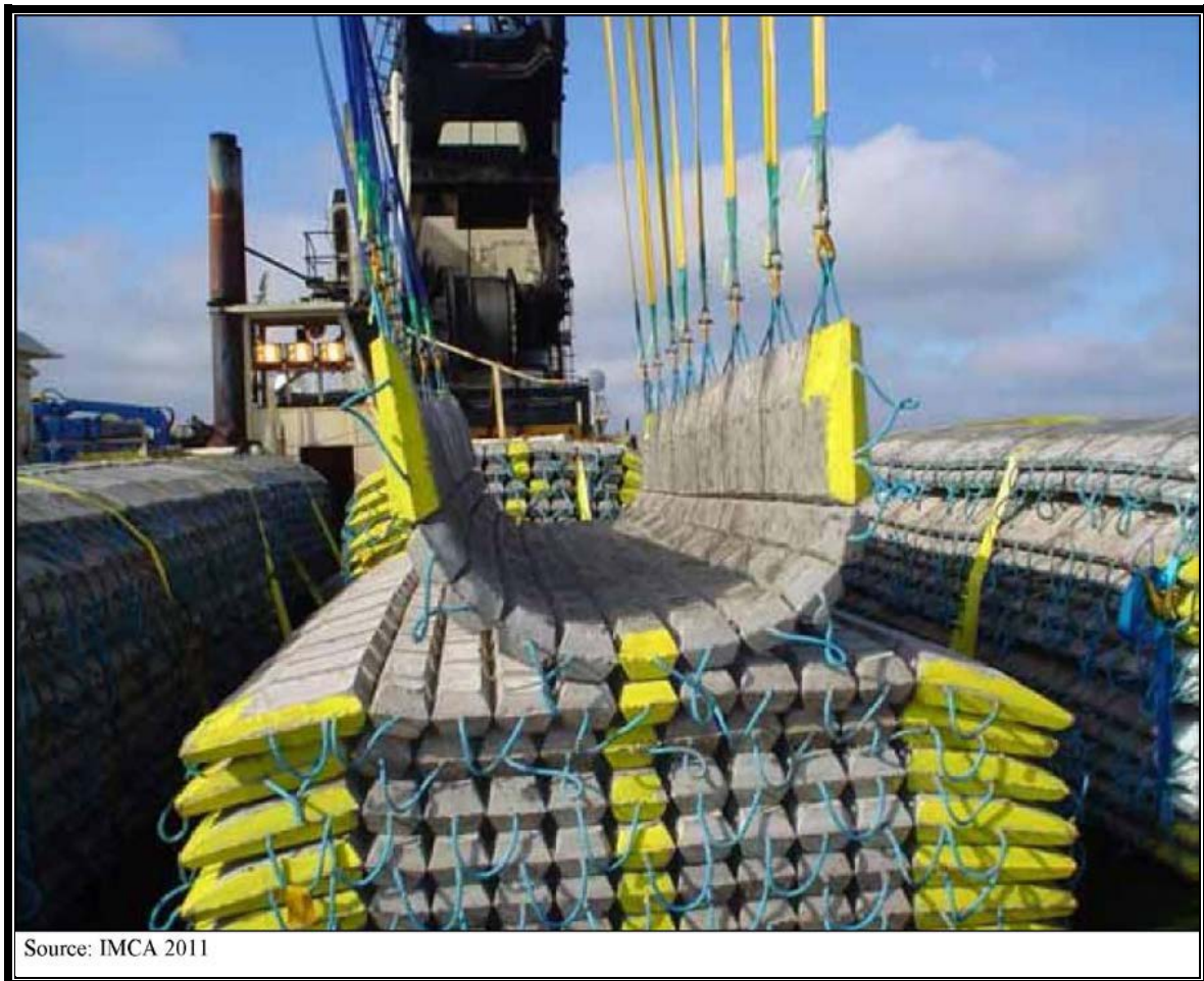
FIGURE 2-5 TYPICAL ARTICULATED CONCRETE MATS
