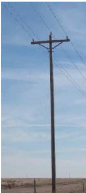
Figure 12. Typical Distribution Line Pole.
