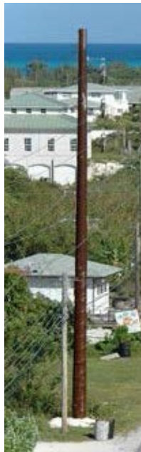
Figure 8. Typical weathered pole.
