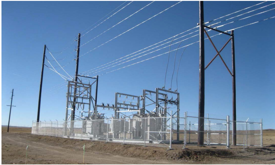
Figure 9. Example of Skid Mounted Substation
