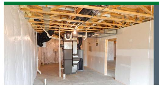
The high-efficiency furnace and heat pump water heater are located in a mechanical room in the insulated, unfinished basement.
