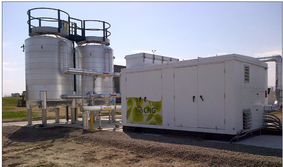
BioCNG purification installation at the Persigo Wastewater Treatment Plant jointly owned by the City of Grand Junction and Mesa County, Colorado. (Photo courtesy of the State Energy Program)
