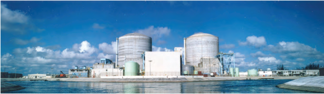
The reactor is surrounded by a massive concrete and steel reinforced containment building 2 to 3 meters (6 to 10 feet) thick. This picture shows the two containment buildings for reactors at St. Lucie plant in Florida.
