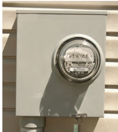
Meters measure a customer's use of electricity so that bills are accurate.
